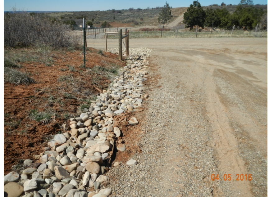
Photo 4: View cobble run-down along the access that appears to be functioning.
