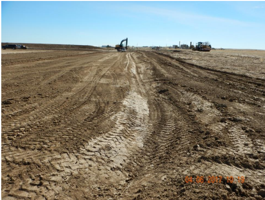
Photo 3. Photo taken from the southwest production area, facing East. Diversion ditch installed in conjunction with a sediment trap.
