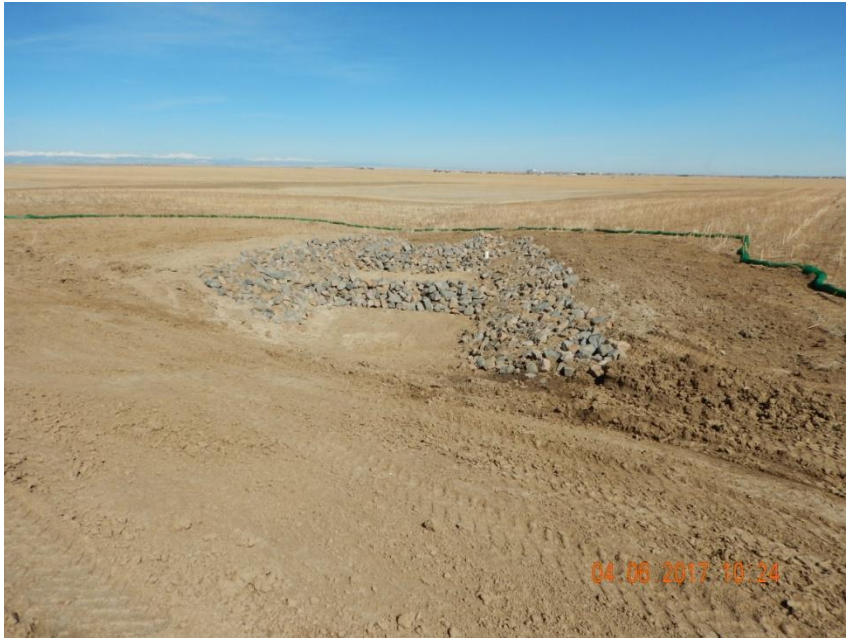
Photo 5. Photo taken from the northwest location, facing Northwest. Sediment trap has been installed in conjunction with diversion ditches and filtrex installed along the outer perimeter of the disturbance area.
