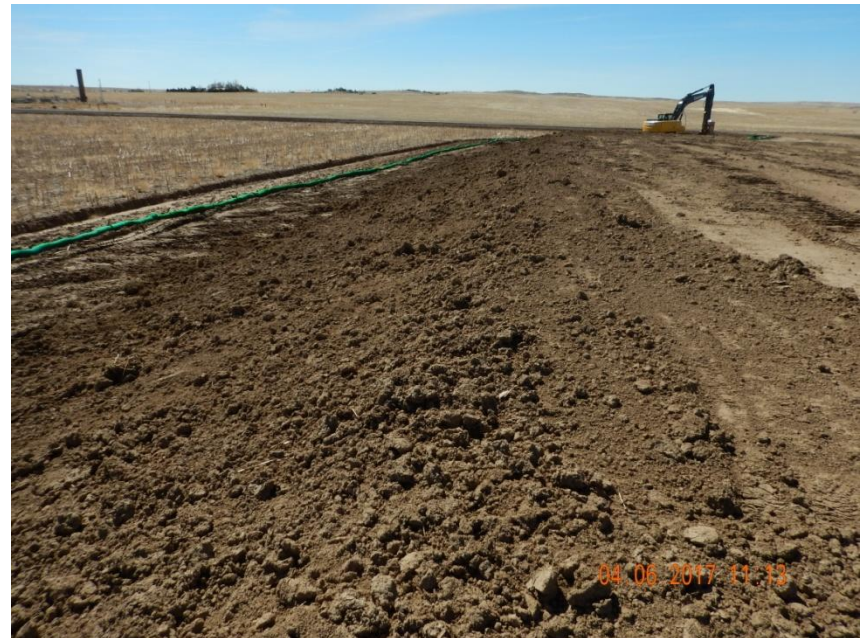
Photo 10. Photo taken from the topsoil stockpile along the eastern location, facing South. Filtrex has been installed along the toe of the topsoil stockpile with a diversion ditch to the outside to control run-on.
