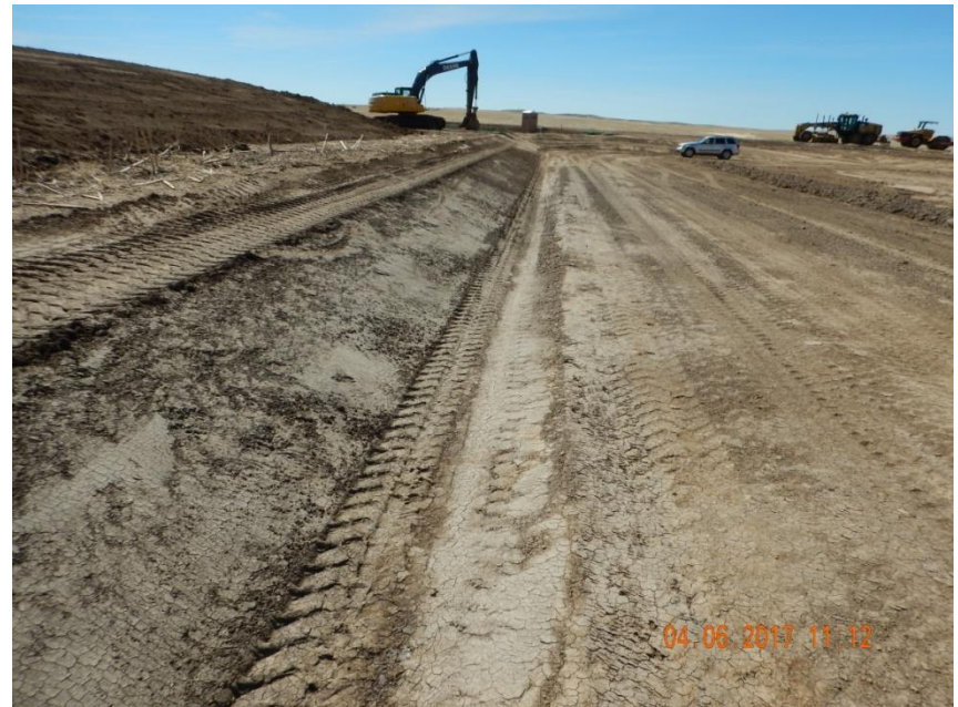
Photo 8. Photo taken from the eastern production area, facing South. Diversion ditch has been installed in conjunction with a sediment trap.
