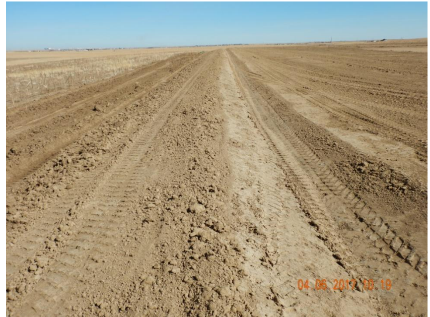
Photo 4. Photo taken from the western production area, facing East. Diversion ditch installed in conjunction with a sediment trap. Operator said that filtrex will be installed along the western disturbance area.
