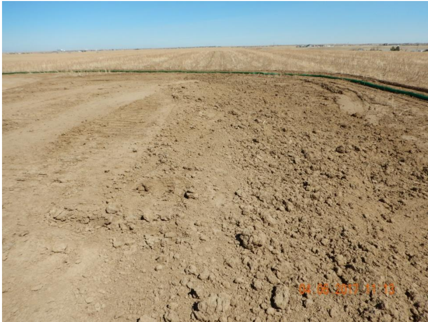
Photo 9. Photo taken from the topsoil stockpile along the eastern location, facing North. Filtrex has been installed along the toe of the topsoil stockpile with a diversion ditch to the outside to control run-on.
