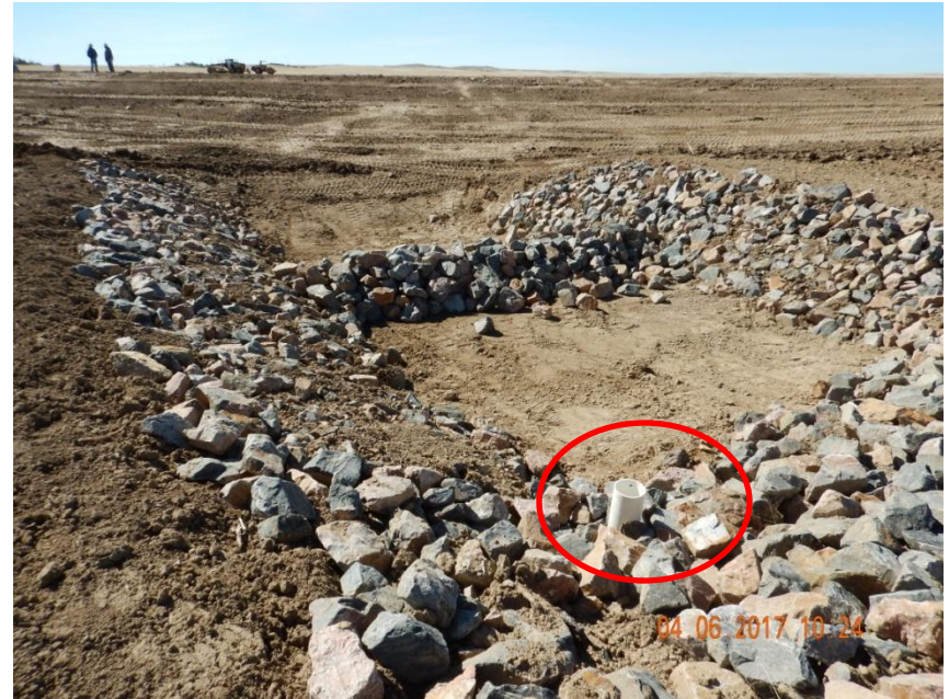
Photo 6. Photo taken from the sediment trap, facing South. Sediment trap has been installed with a stabilized outfall and principle outlet.
