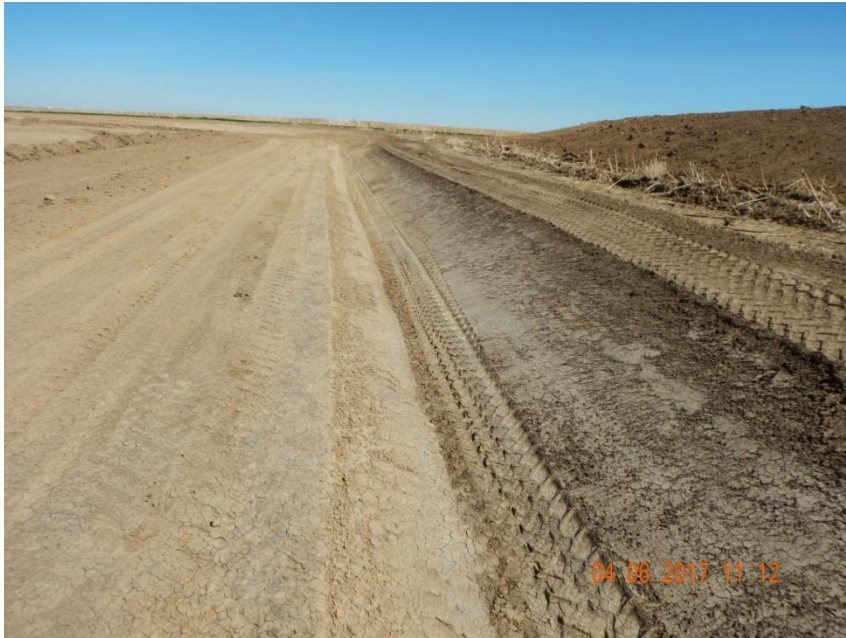
Photo 7. Photo taken from the eastern production area, facing North. Diversion ditch has been installed in conjunction with a sediment trap.
