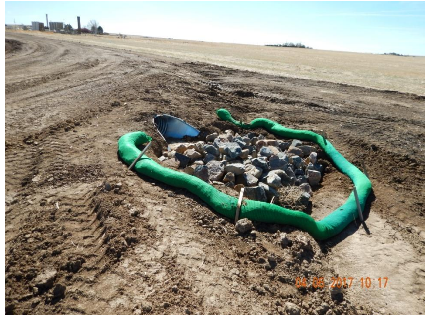
Photo 2. Photo taken from the southeast location, facing Southeast. A stabilized outlet has been installed with a filter wattle.
