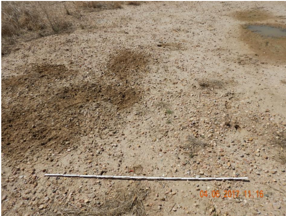
Photo 4: Photo taken from the location. Photo shows large portions of the location where gravel and base material have not been removed and remain unvegetated. 6 foot measuring stick for reference.
