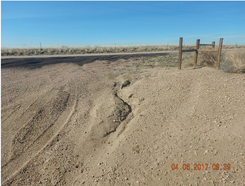
Photo 3: Stormwater erosion on SW corner of location, looking SW
