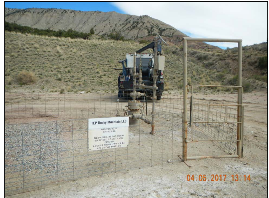
Wireline unit rigging down after replacing stankding valve in well.
