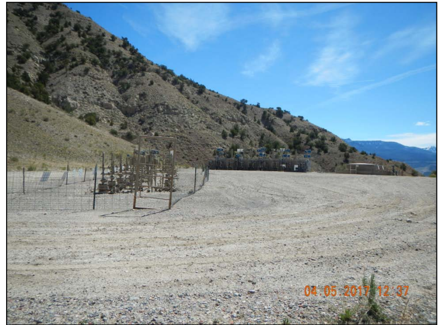
Facility tank and equipment.
