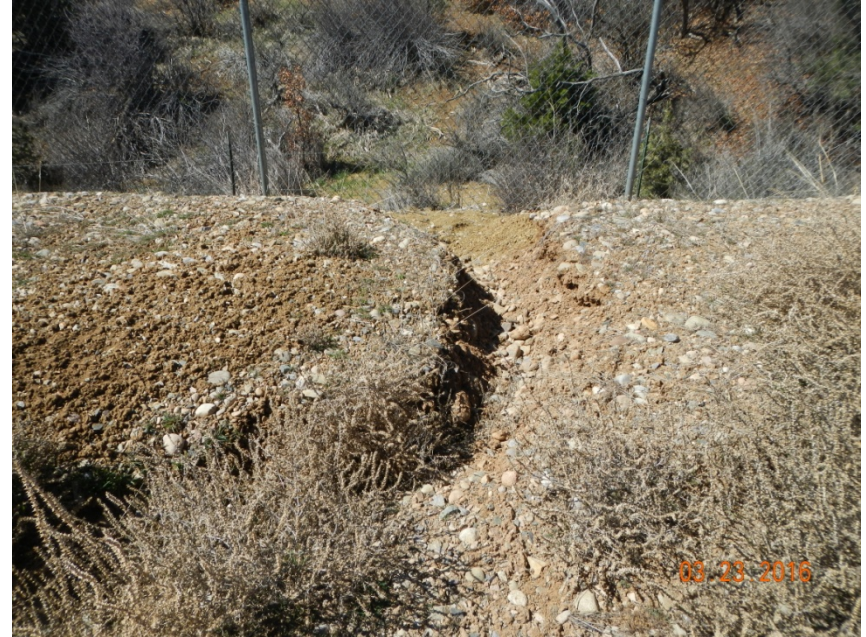
Photo 6: View of erosional channel (approximately 2 feet wide and deep) forming within the western portion of the project area.
