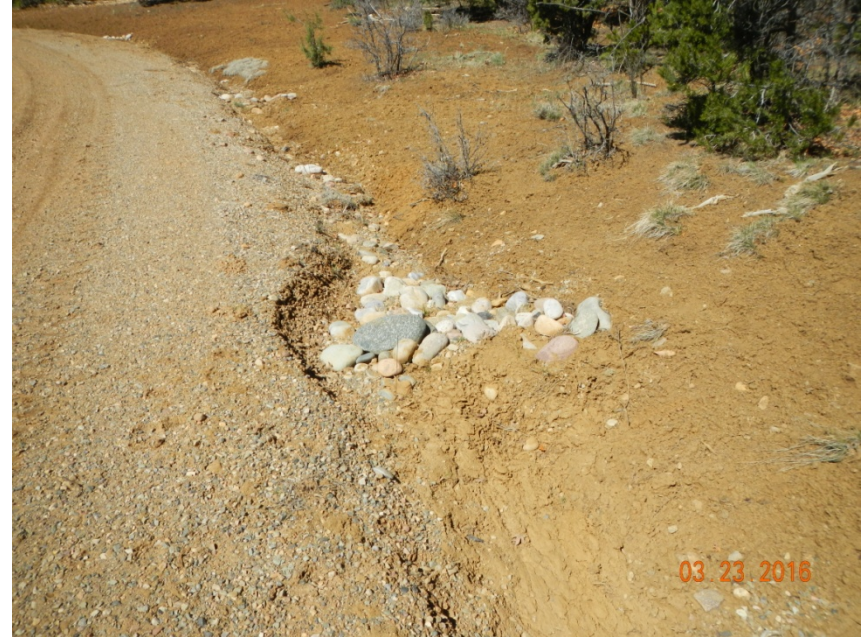
Photo 6: View of cobble check dam along the access road that is full of sediment and eroding where stormwater flows around the dam.
