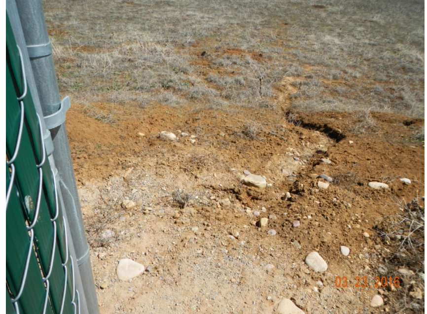
Photo 6: View of erosional channels in the southeastern corner of the project area.
