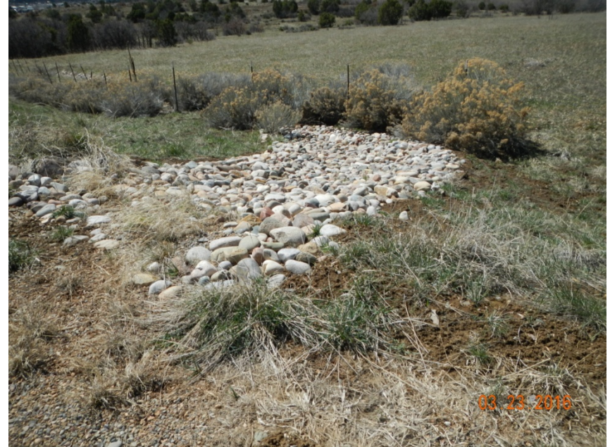
Photo 6: View of stormwater controls in the western portion of the project area appear to be functioning.
