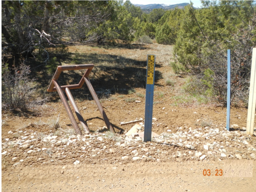
Photo 9: View of pipe barricade that looks like it's been knocked over.
