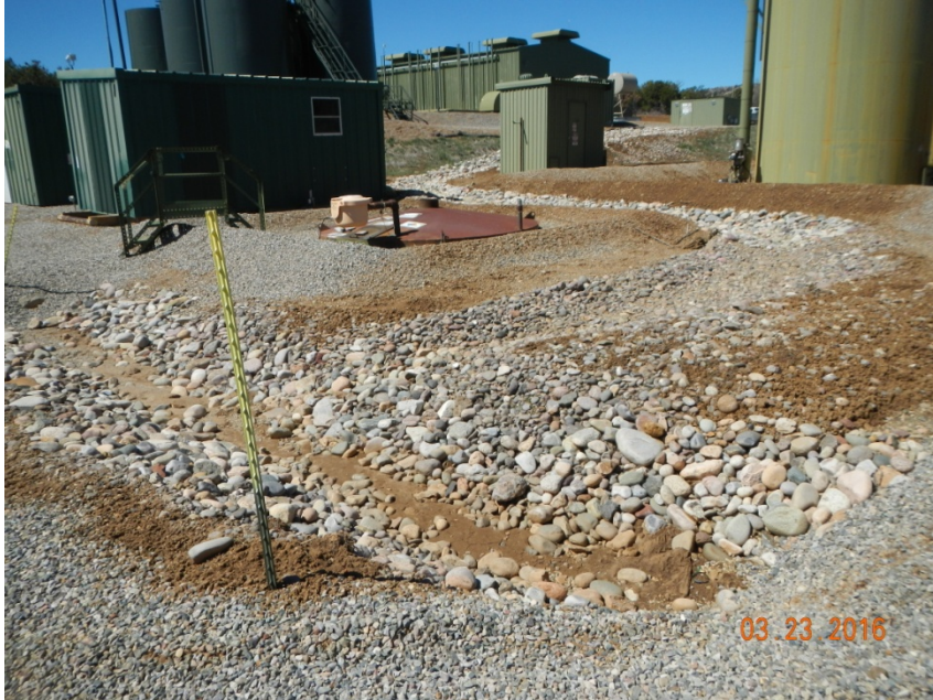
Photo 7: View of stormwater management in the northwestern portion of the project area that appears to be functioning.
