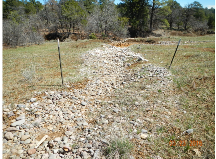
Photo 6: View of stormwater controls and drainage to a silt trap at the edge of the project area.
