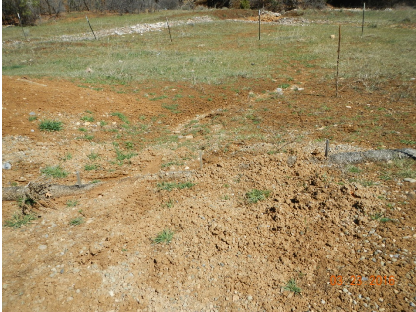
Photo 5: View of wattles in the eastern portion of the project area that are not functioning.
