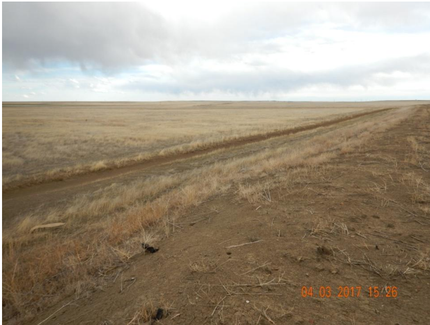
Photo 7. Photo taken from the eastern location, facing Southeast. A ditch and berm BMP has been installed around the location perimeter. Minor rill erosion was observed along the fill slopes.
