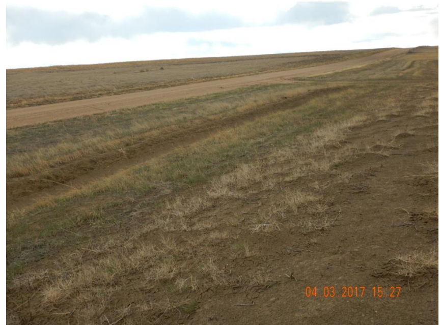
Photo 8. Photo taken from the southern location, facing Southwest. A ditch and berm BMP has been installed around the location perimeter. Minor rill erosion was observed along the fill slopes.
