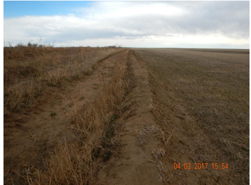
Photo 6. Photo taken of the southwestern location, facing South. Berm BMP has been repaired and built up higher.
