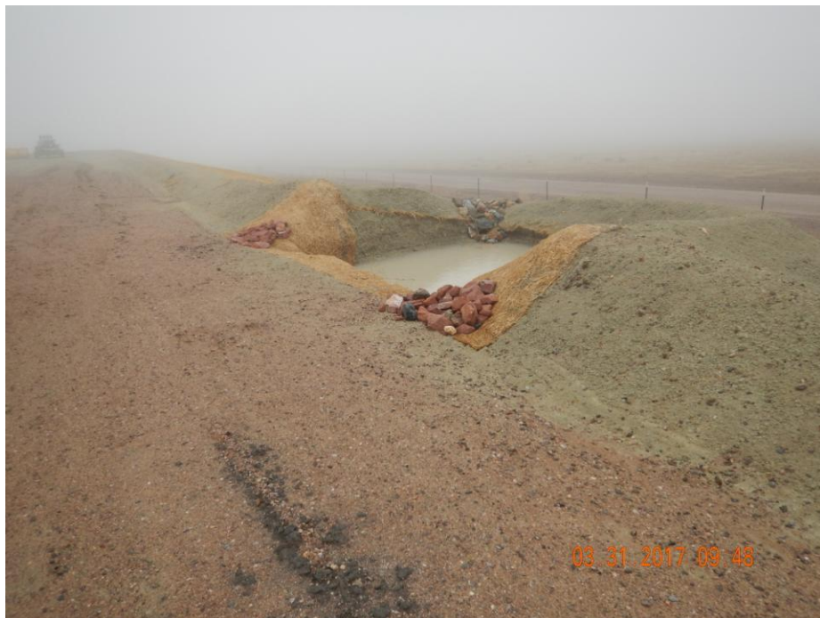
Photo 1: Photo taken from the north end of the location, facing west. Photo shows additional inlet protection has been installed on sediment trap.
