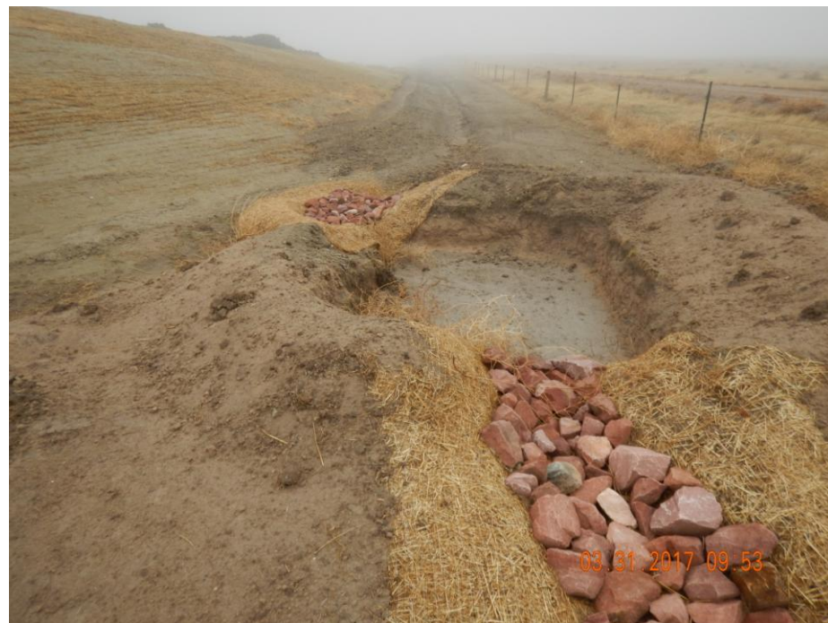
Photo 6: Photo taken from the southwest corner of the location, facing east. Photo shows a stormwater and sediment trap has been constructed on this corner of the location. Trap appears to be in proper functioning condition.
