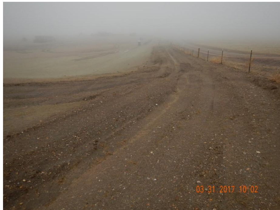
Photo 10: Photo taken from the northeast corner of the location, facing west. Photo shows example of an area of ditch with long stretches of downward slope without controls to mitigate stormwater velocity.
