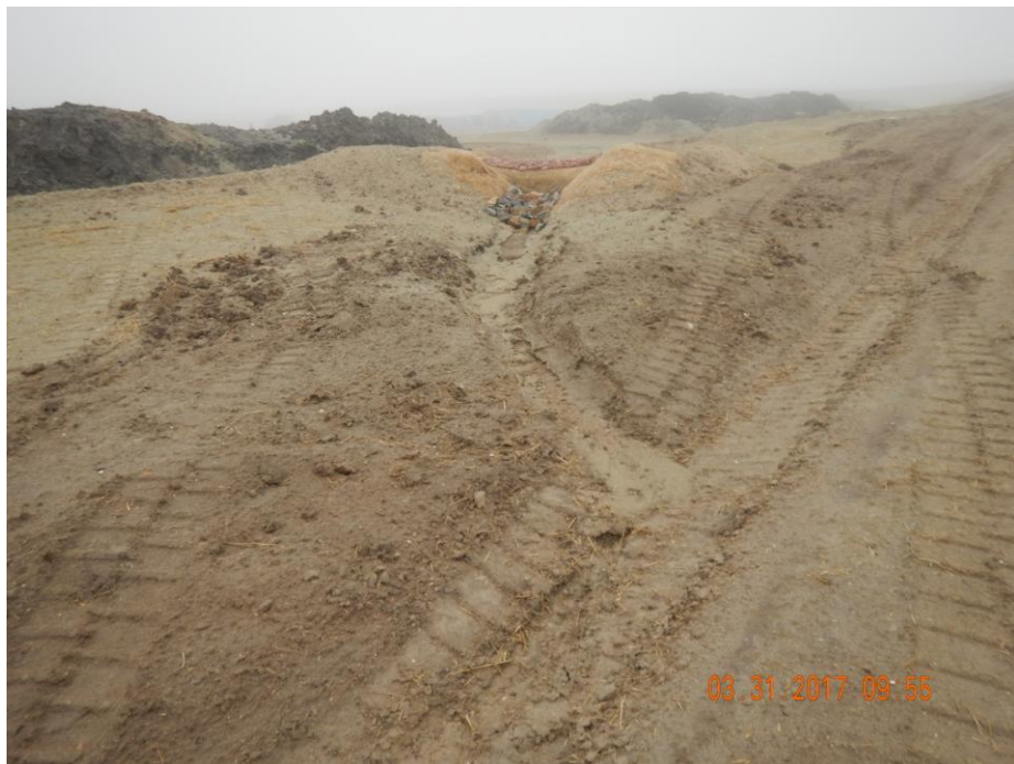
Photo 7: Photo taken from the outlet of the sediment trap on the south end of the location. Photo shows that outlet armoring appears insufficient as stormwater erosion leading into the ditch is evident.
