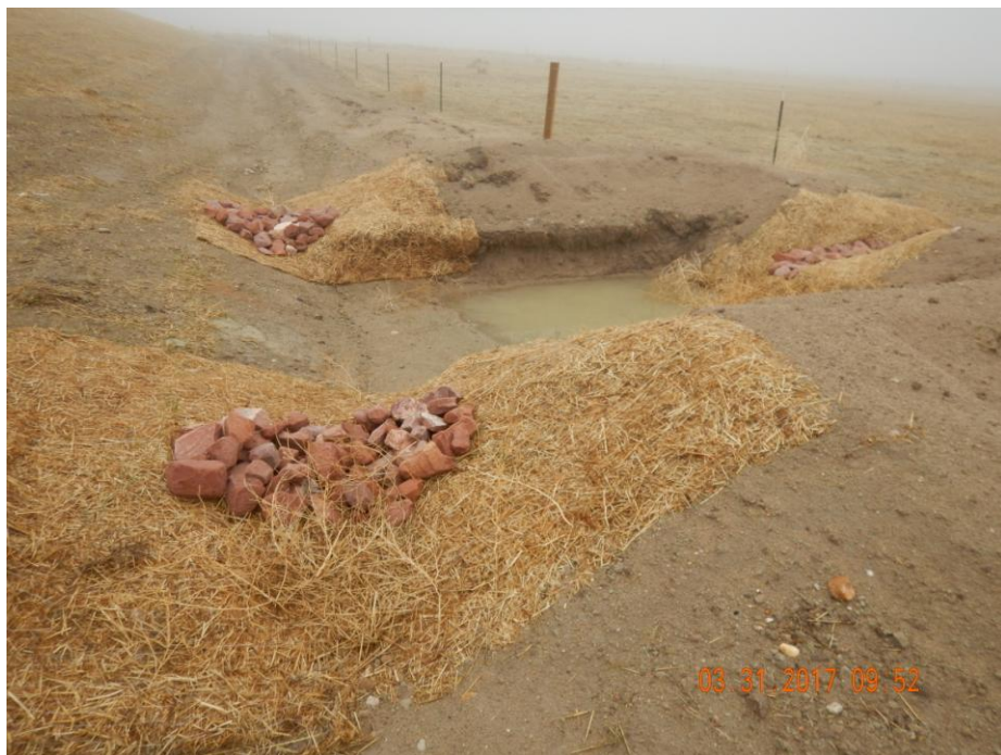
Photo 5: Photo taken from the northwest end of the location. Photo shows that additional inlet and outlet protection has been installed on the sediment traps.
