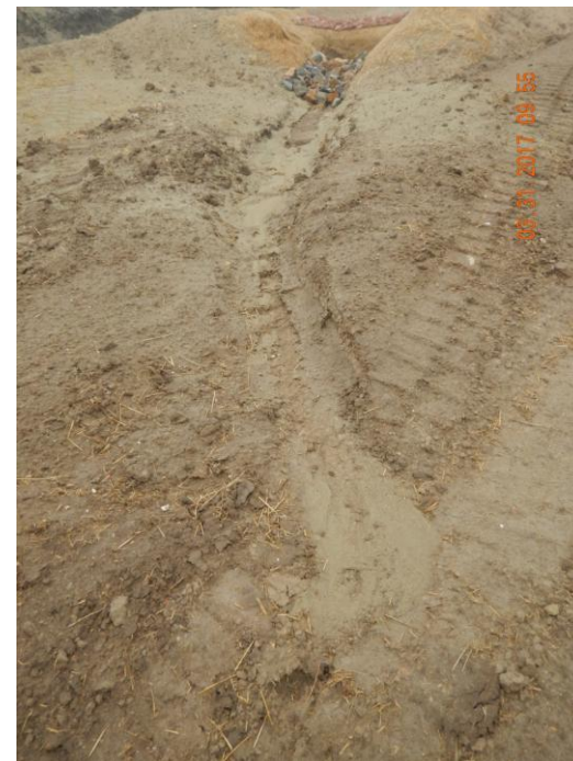
Photo 8: Photo taken from the outlet of the sediment trap on the south end of the location. Photo shows that outlet armoring appears insufficient as stormwater erosion leading into the ditch is evident.
