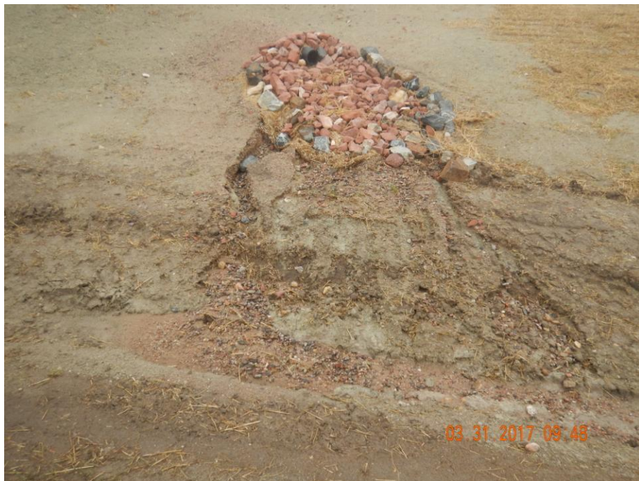
Photo 3: Photo taken from the outlet of the sediment trap on the north end of the location. Photo shows that outlet armoring from the drain was insufficient as stormwater erosion leading into the ditch is evident.
