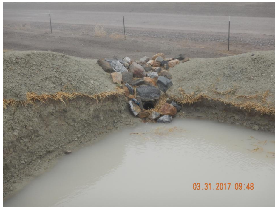
Photo 2: Photo taken from the north end of the location. Photo shows additional outlet drain constructed into sediment trap.
