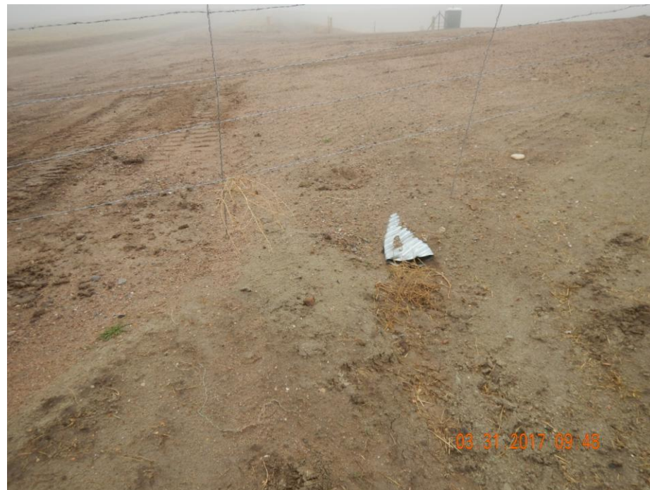
Photo 4: Photo taken from the access road on the north end of the location. Photo shows culvert has been smashed and in need of maintenance.
