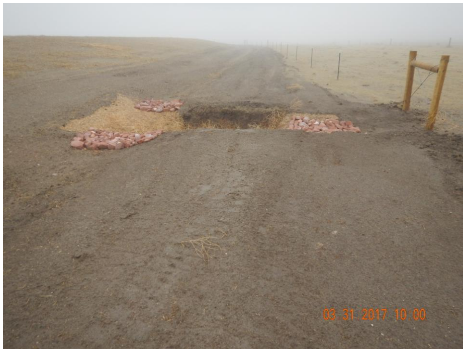
Photo 9: Photo taken from the east end of the location. Photo shows additional inlet and outlet protection has been installed on sediment trap.
