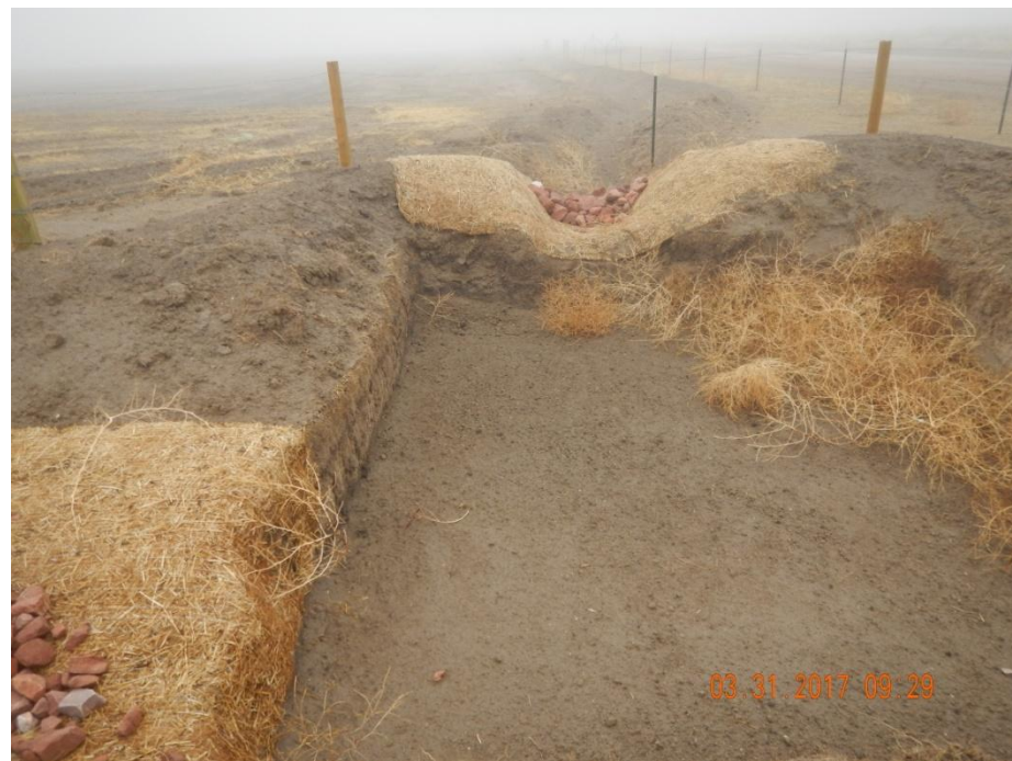
Photo 3: Photo taken from the northwest end of the location, facing south. Photo shows sediment trap has had additional inlet and outlet protection implemented and appears to be sufficient and in proper functioning condition.
