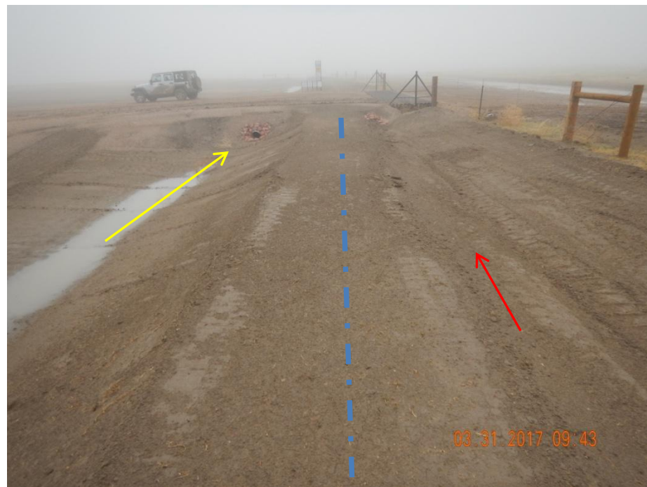
Photo 8: Photo taken from top of berm (blue line) between ditch on the north end of the location and the pad. Arrow in yellows shows likely stormwater flow and ponding once sediment trap has reached capacity. Red arrow represents stormwater flow within ditch.
