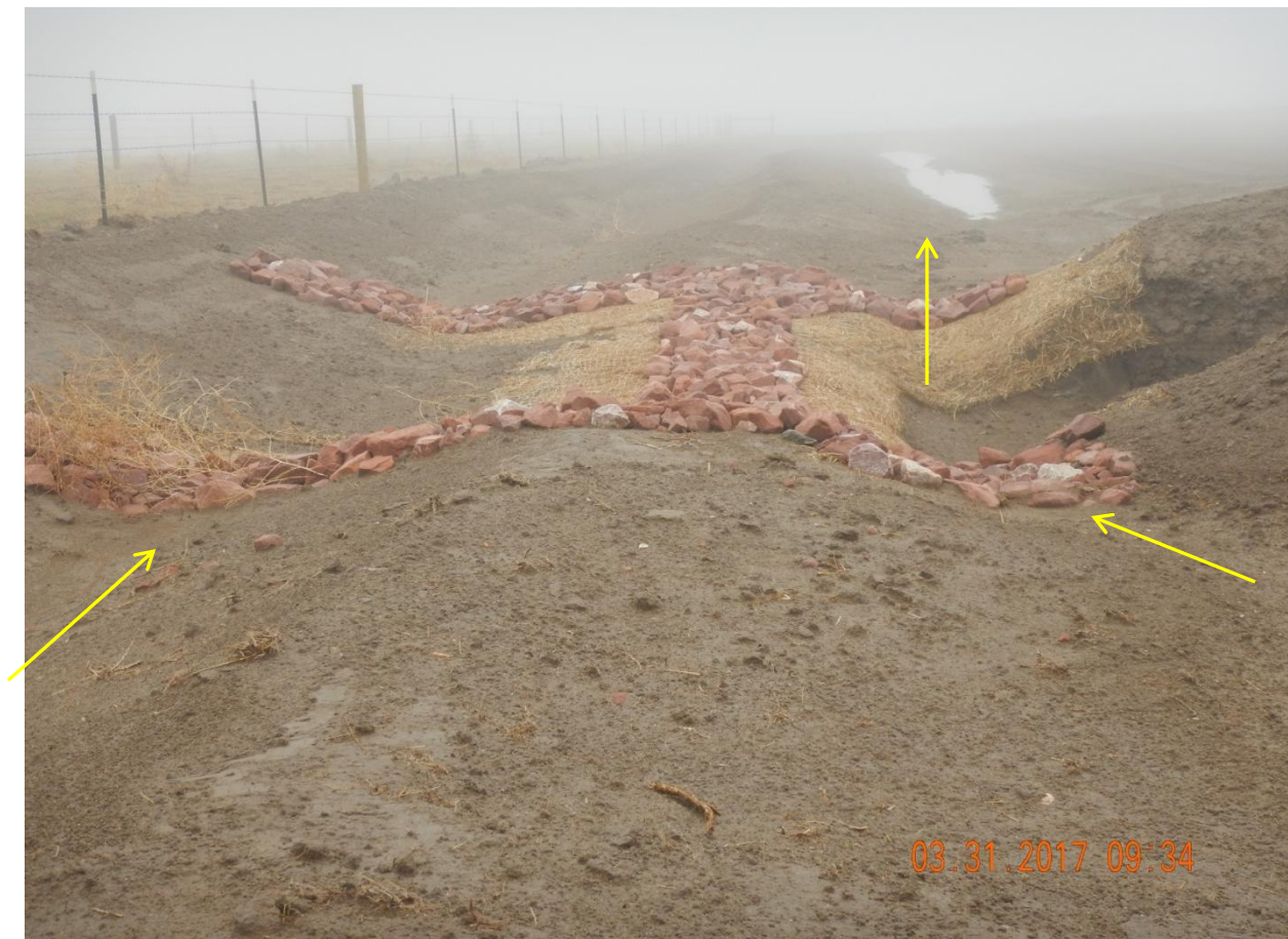
Photo 4: Photo taken from the south end of the location facing west. Photo shows sediment trap has had additional inlet and outlet protection implemented, however trap has been constructed in such a manner that stormwater would more likely flow from the ditch into the trap, rather than the trap into ditch. Also, it appears once trap has reached capacity, stormwater will likely flow out onto the location and pond to the west. Stormwater flow represented by yellow arrows. Trap does not appear to have been constructed with proper planning or good engineering practices to protect the site during inclement weather conditions
