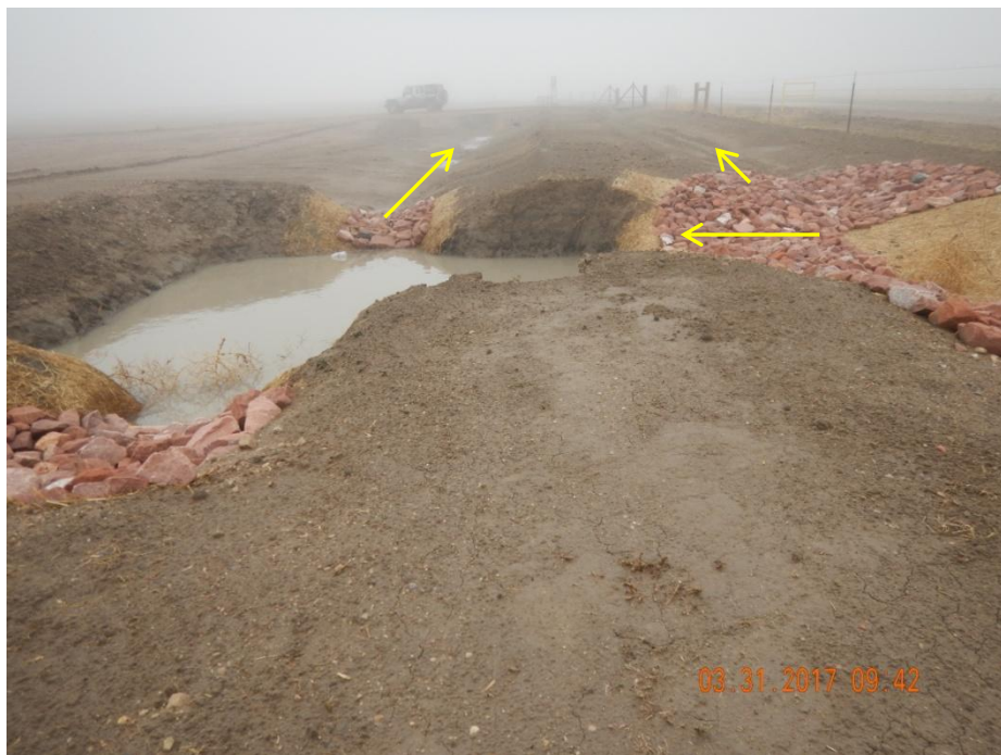
Photo 7: Photo taken from sediment trap on the north end of the location, facing west. Photo shows trap appears to have been constructed in such a manner that stormwater would more likely flow from the ditch into the trap, rather than the trap into ditch. It also appears once trap has reached capacity, stormwater will likely flow out onto the location and pond to the west. Stormwater flow represented by yellow arrows
