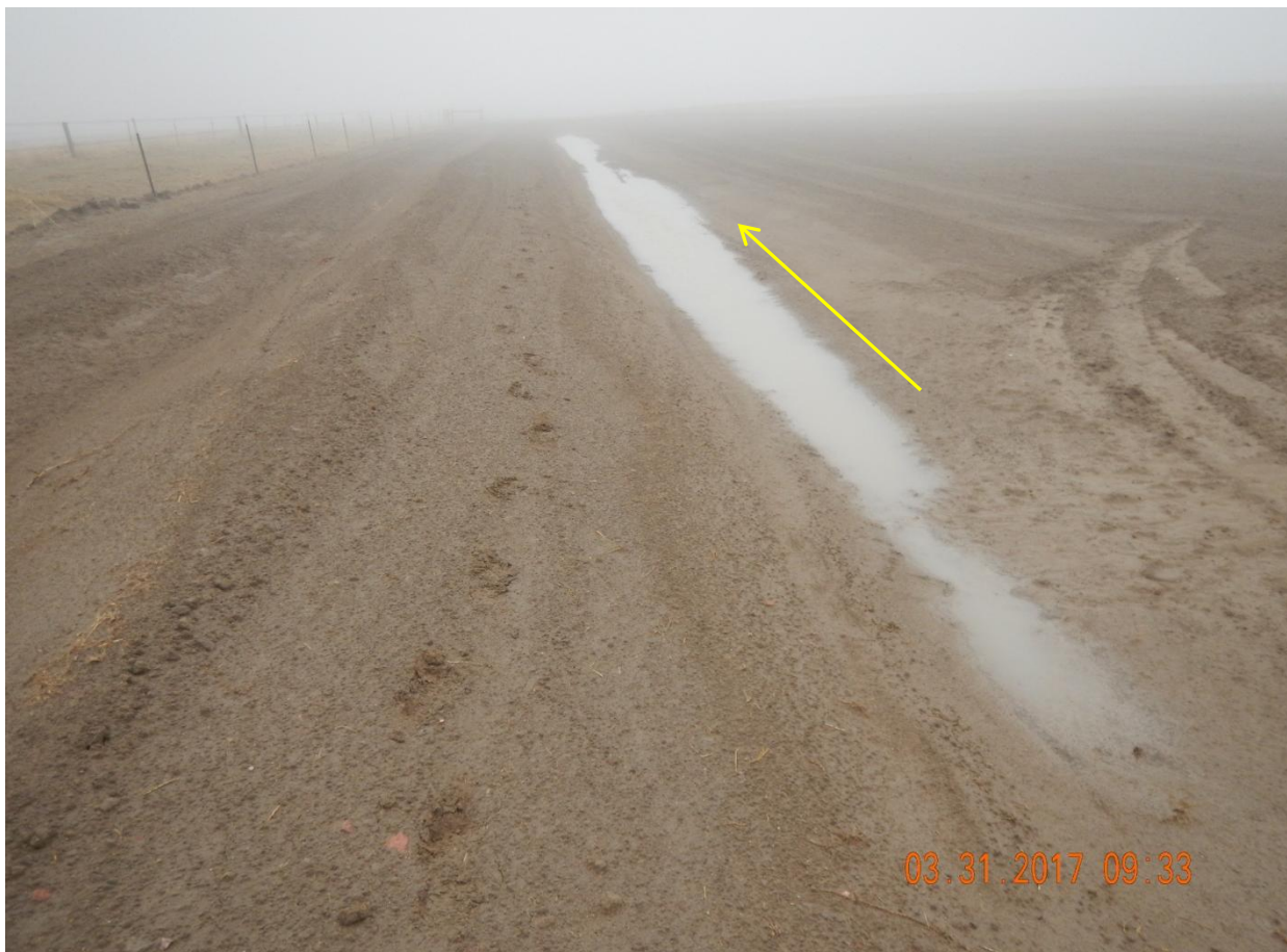
Photo 5: Photo taken to the west of the sediment trap seen in photo 4. Photo shows area on the southwest end of the location where water appears to concentrate and pond. Once trap has reached capacity, stormwater will likely flow out onto the location and pond here.
