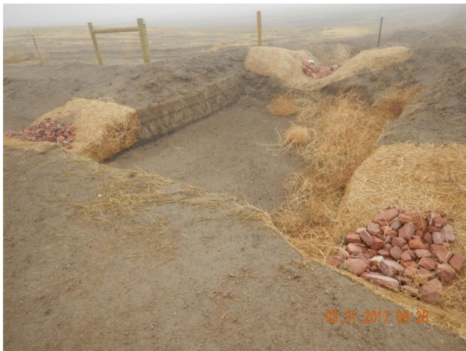
Photo 2: Photo taken from the northwest end of the location, facing south. Photo shows sediment trap has had additional inlet and outlet protection implemented and appears to be sufficient and in proper functioning condition.
