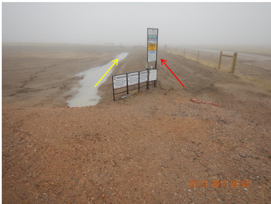
Photo 9: Photo taken access road above the culvert seen in photo 8.(blue line) on the north end of the location and the pad. Arrow in yellow shows area of stormwater flow and ponding once sediment trap has reached capacity. Red arrow represents stormwater flow within ditch.
