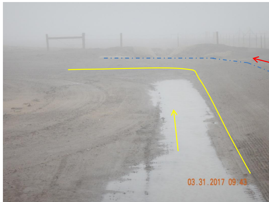
Photo 10: Photo taken from the northwest end of the location, facing west. Photo shows areas (yellow arrow/line) of stormwater flow and ponding once sediment trap has reached capacity. Red arrow represents stormwater flow within ditch. Berm separating stormwater ditch and pad represented by blue line.
