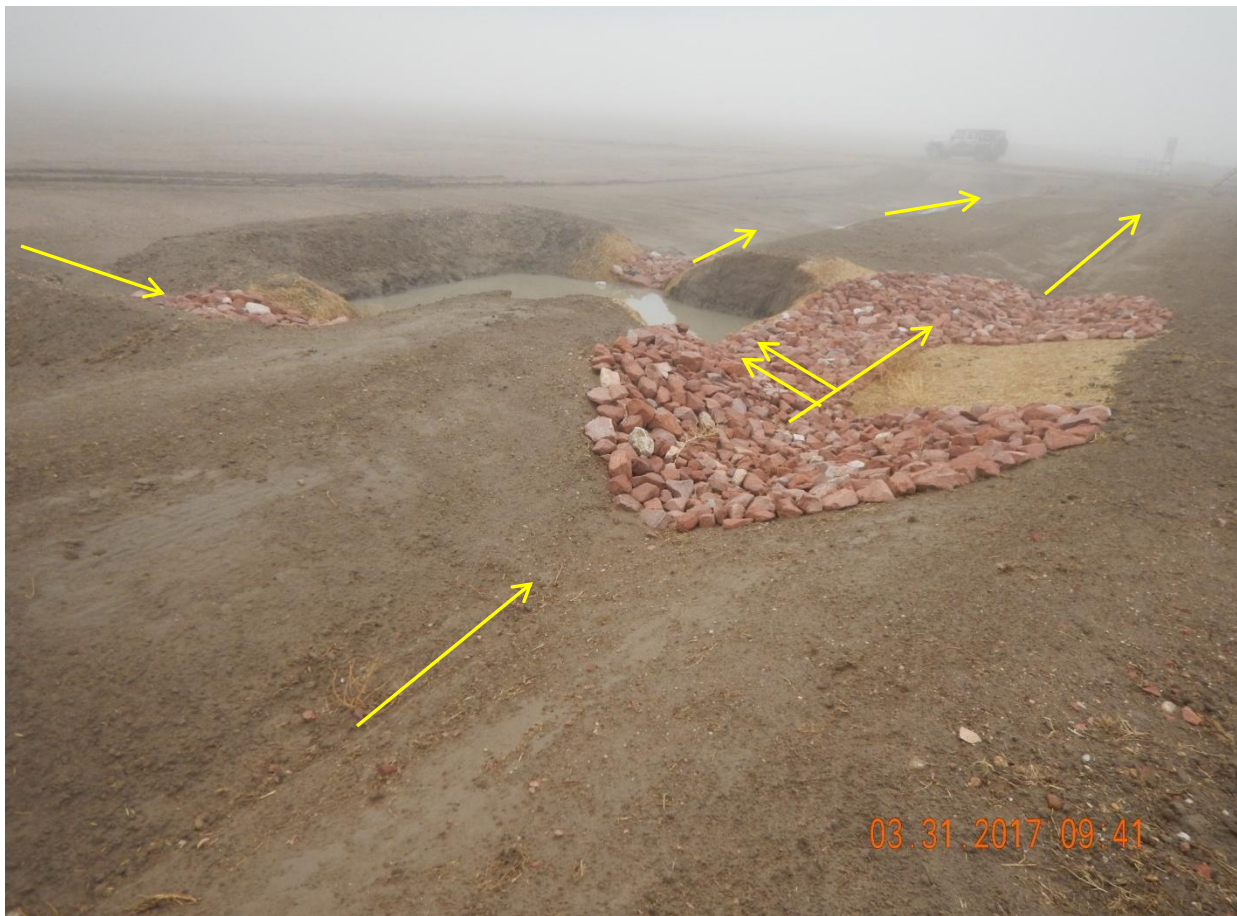
Photo 6: Photo taken from the north end of the location facing west. Photo shows sediment trap has had additional inlet and outlet protection implemented, however trap has been constructed in such a manner that stormwater would more likely flow from the ditch into the trap, rather than the trap into ditch. Also, it appears once trap has reached capacity, stormwater will likely flow out onto the location and pond to the west. Stormwater flow represented by yellow arrows. Trap does not appear to have been constructed with proper planning or good engineering practices to protect the site during inclement weather conditions
