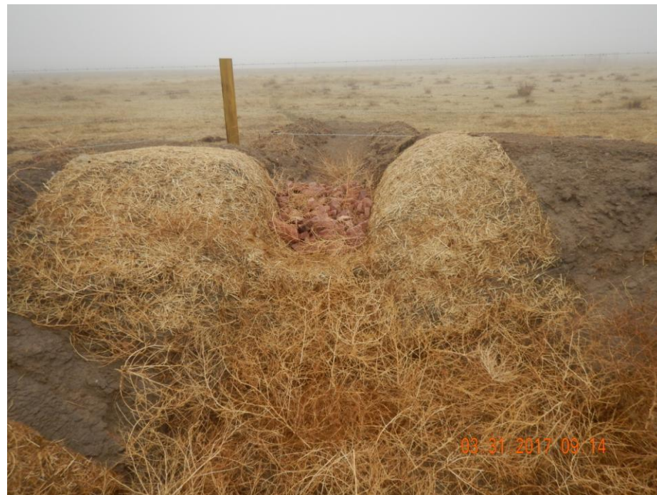
Photo 2: Photo taken from the west end of the location, facing west. Photo shows sediment trap has had additional inlet and outlet protection implemented and appears to be sufficient and in proper functioning condition.
