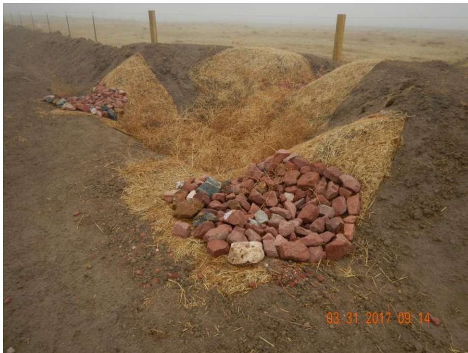
Photo 1: Photo taken from the west end of the location, facing west. Photo shows sediment trap has had additional inlet and outlet protection implemented and appears to be sufficient and in proper functioning condition.
