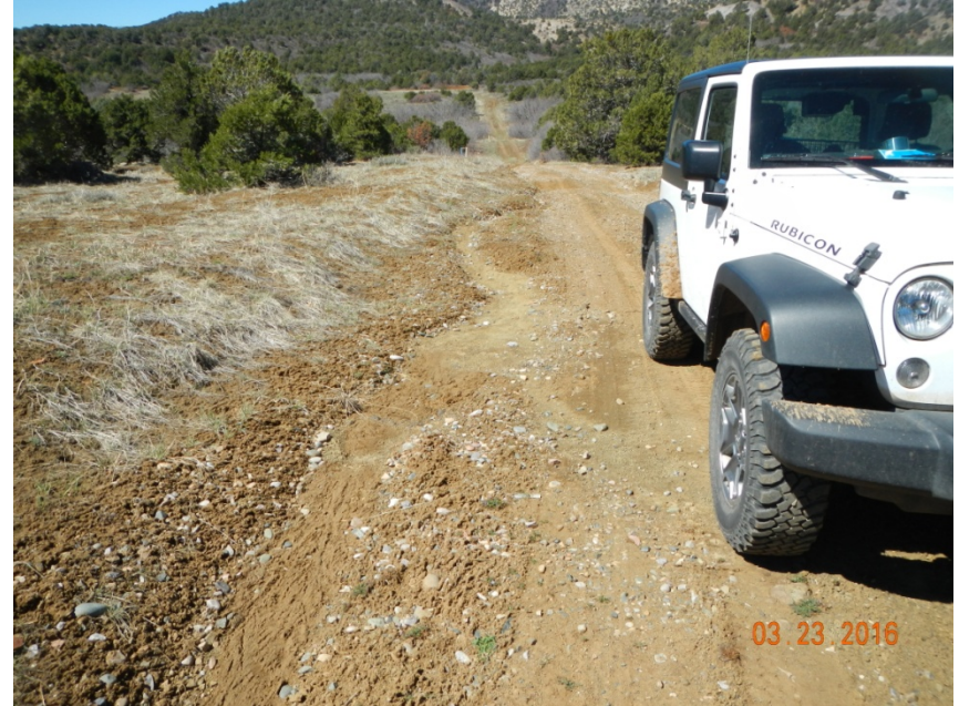
Photo 6: View of area along the access road where concentrated stormwater flows are eroding the sides of the access road.
