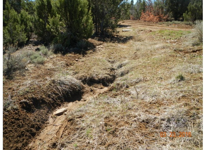
Photo 4: View of area downstream from culvert near the entrance to the well pad where a head-cut is forming. This area needs to be stabilized.
