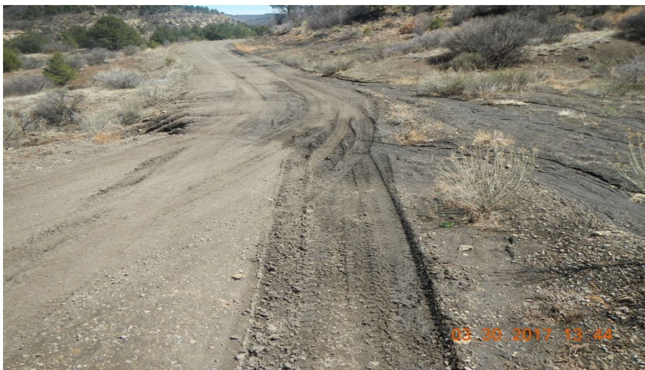
photo 2: Facing southeast, erosion occurring in photo 1 is depositing sediment in this area and stormwater is flowing across the road causing erosion.
