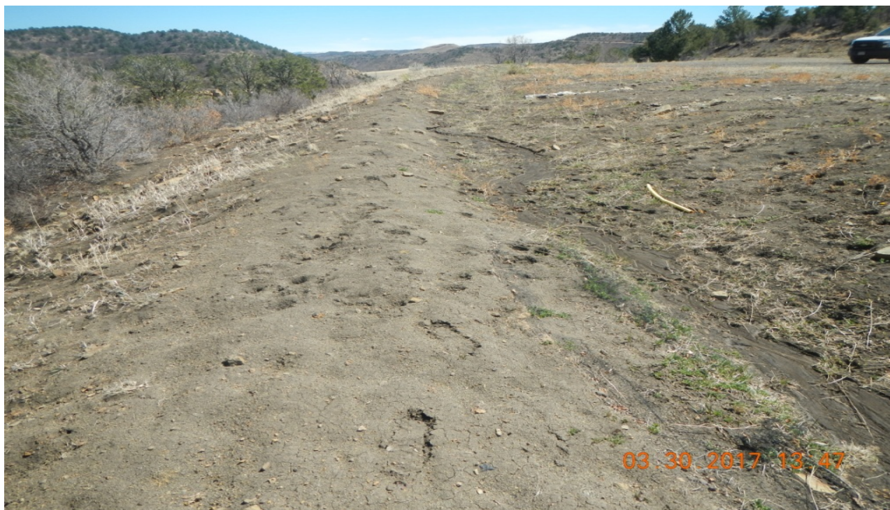
photo 5: Facing southeast at the location. There are areas where vegetation has not established and soils are not stabilized.
