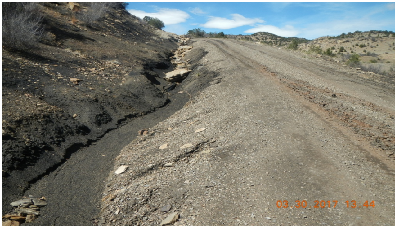
photo 1: Facing northwest, there are signs of erosion occurring along the side of the access road.
