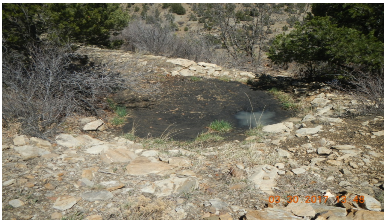
photo 6: Sediment trap at the east side of the location is full of sediment.
