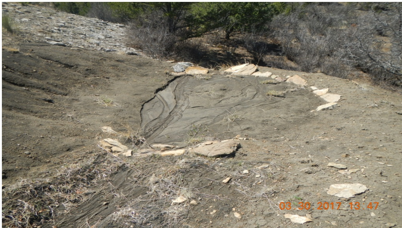
photo 4: The sediment trap at the northwest side of the location is full of sediment.
