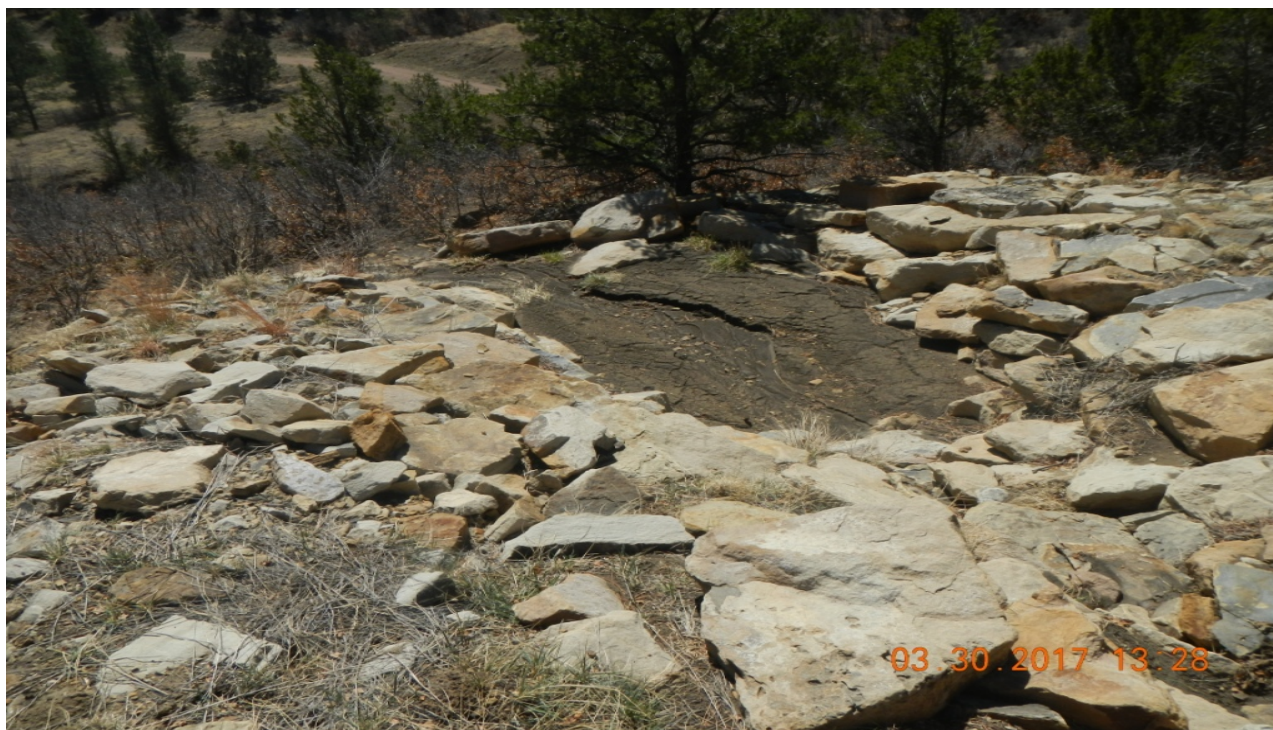
photo 3: The sediment trap is full of sediment at the southwest side of the location.
