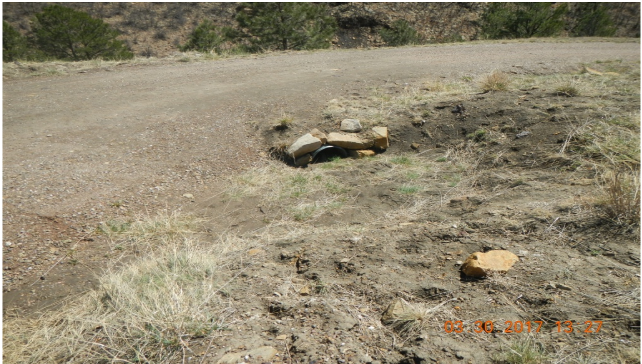
photo 1: The culvert at the location is half full of sediment.
