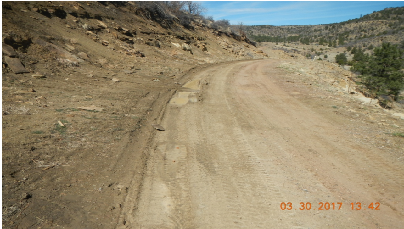
photo 1: There is sediment migration onto the access road.
