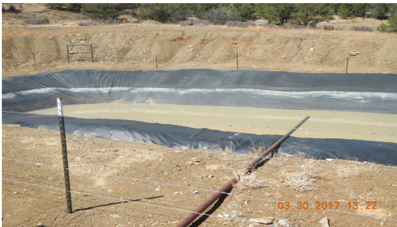
photo 4: Facing toward the pit. Did not notice a freeboard marker.
