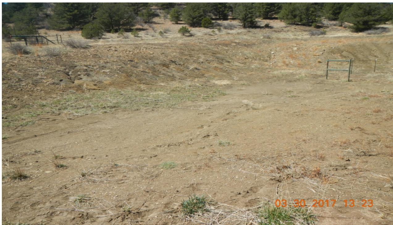
photo 3: Facing toward the west side of the location. There are signs of stormwater run on which is depositing sediment onto the location.
