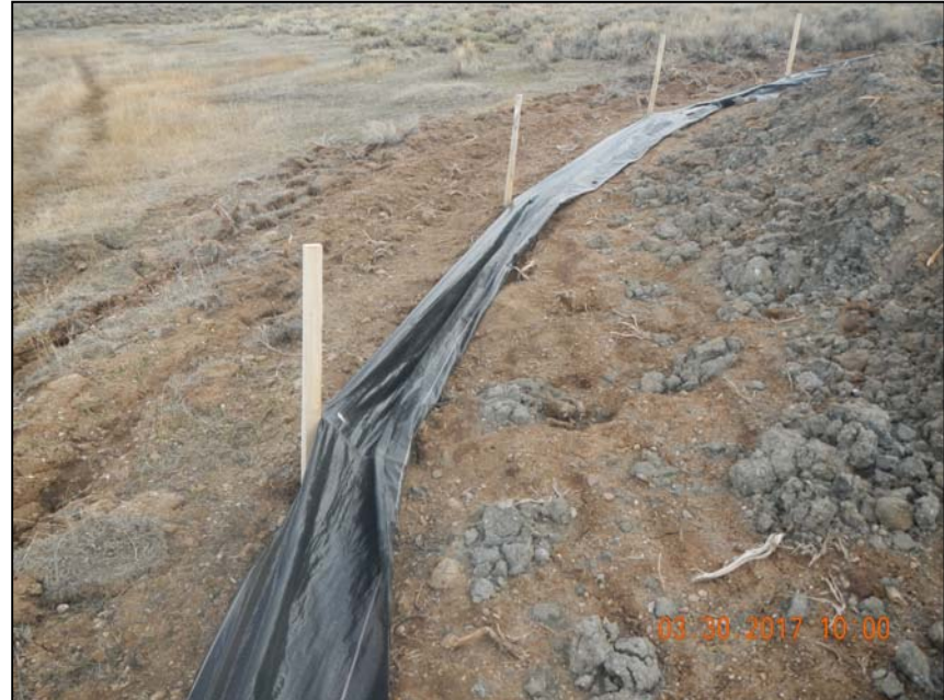
Photo 4. One of many places where silt fence has fallen down.
