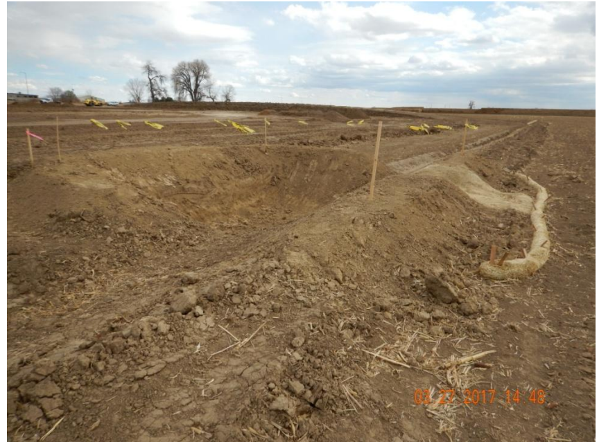
Photo 6. Photo taken from the western location, facing South. Sediment trap installed with outlet protection in the form of a blanket and wattle.
