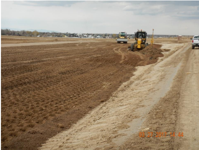
Photo 3. Photo taken from the southeast location, facing North. Cut slope appears to be temporarily stabilized but may need additional BMPs.
