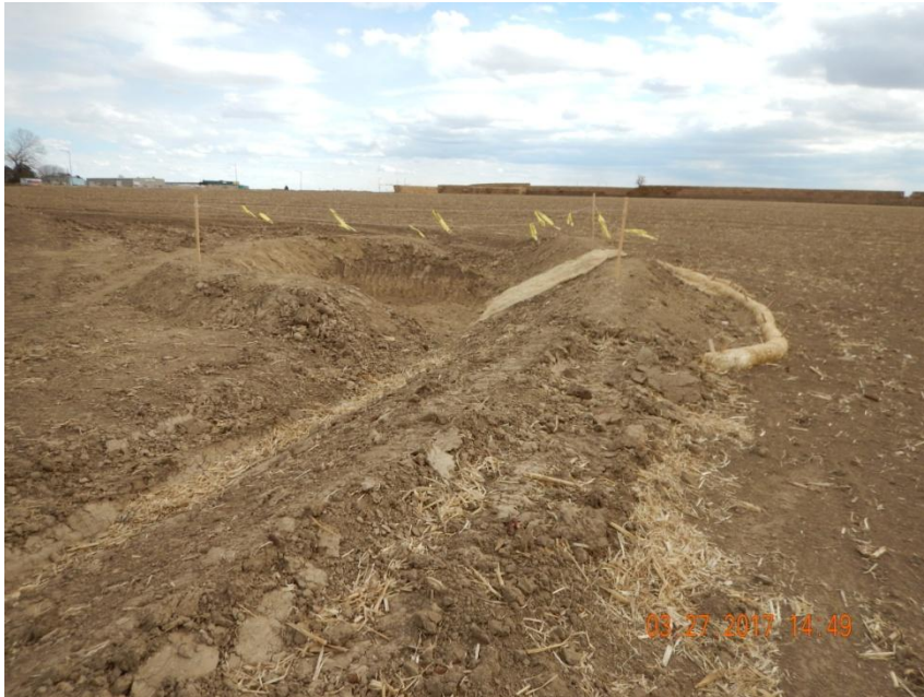
Photo 7. Photo taken from the southwest location, facing South. Sediment trap installed with outlet protection in the form of a blanket and wattle.
