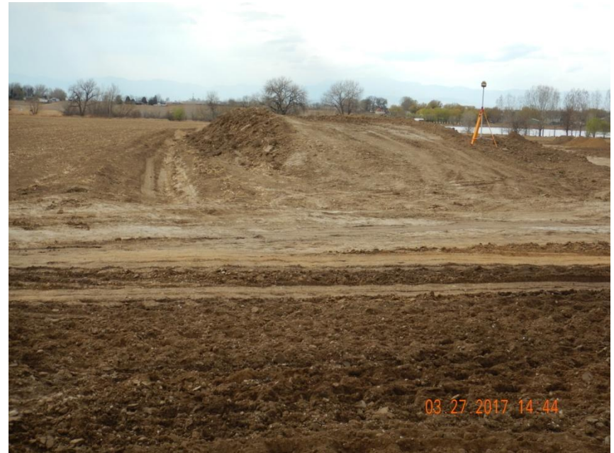
Photo 2. Photo taken from the southeast location, facing West. Ditch and berm BMP installed around north, west, and south perimeter of location. Topsoil stored along the southern perimeter of location.
