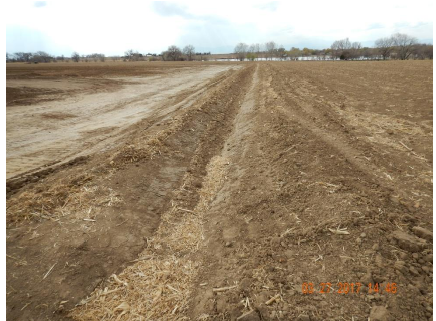
Photo 4. Photo taken from the northern location, facing West. Ditch and berm BMP installed around north, west, and south perimeter of location.
