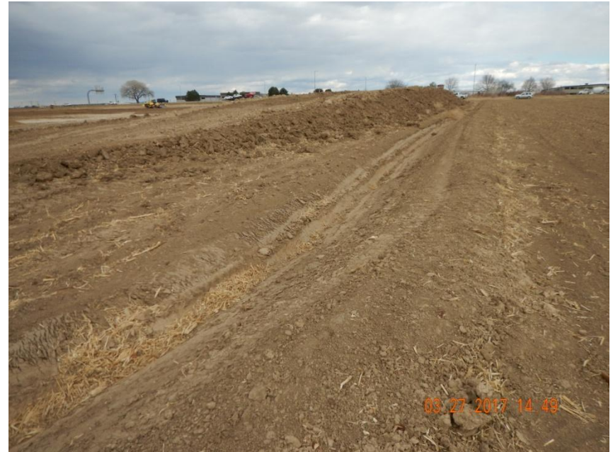
Photo 8. Photo taken from the southern location, facing East. Ditch and berm BMP installed around north, west, and south perimeter of location.
