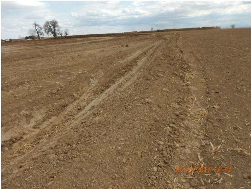
Photo 5. Photo taken from the northwest location, facing South. Ditch and berm BMP installed around north, west, and south perimeter of location.
