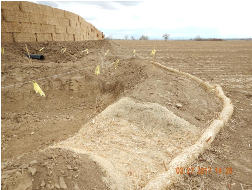
Photo 7. Photo taken from the northwest location, facing South. Sediment trap installed with outlet protection in the form of a blanket and wattle.
