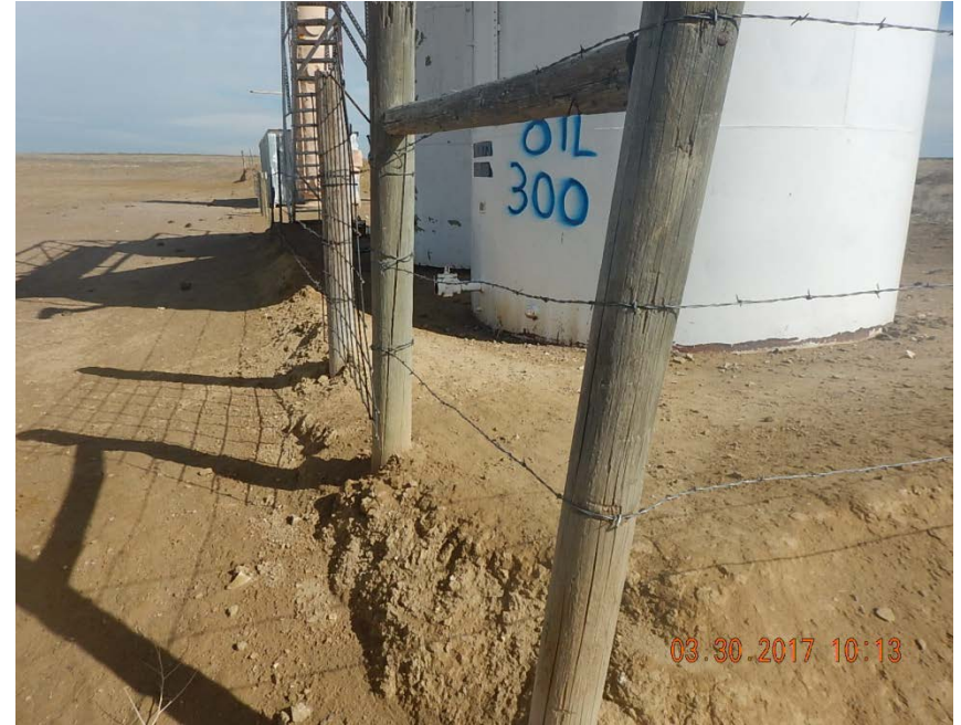
Photo 1: Berms low to nonexistent
