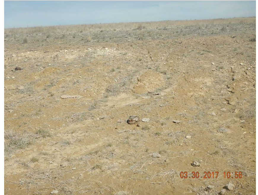
Photo 8: Stormwater erosion on N side of location, looking N
