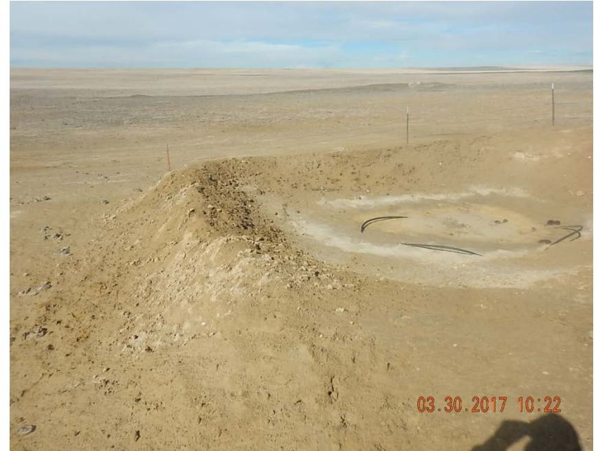
Photo 13: Pit wall built up, 2+ feet of freeboard
