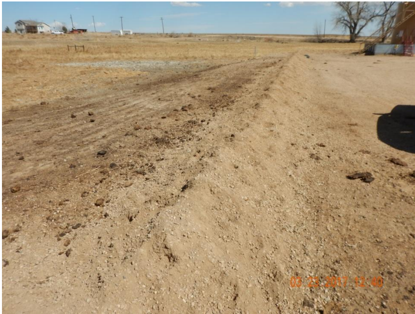
Photo 1. Photo taken from the northern battery location, facing East. An unconsolidated berm has been installed along the north and east production area. Cattle have diminished the quality of the berm along major portions.
