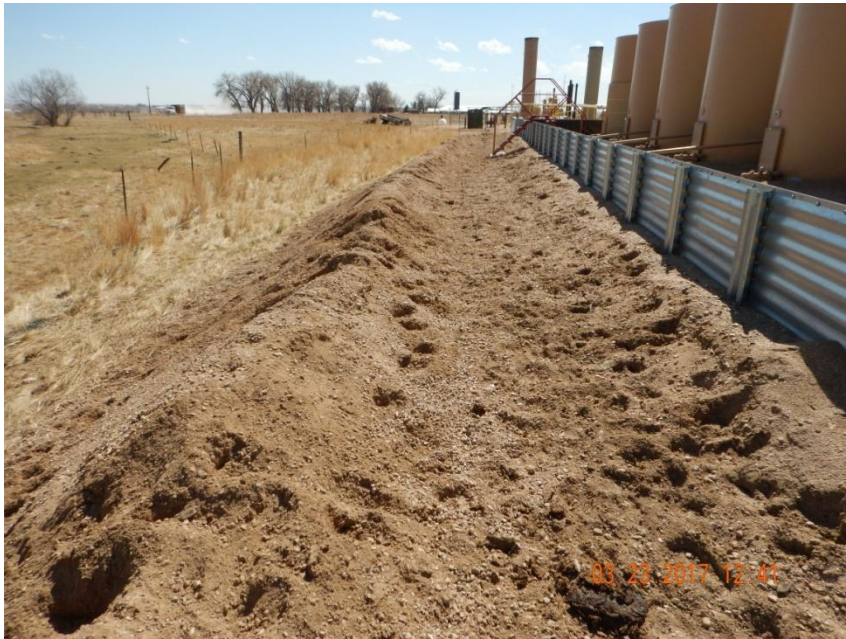
Photo 3. Photo taken from the eastern battery location, facing South. An unconsolidated berm has been installed along the north and east production area. Cattle have diminished the quality of the berm along major portions.
