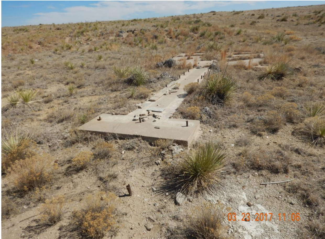
Photo 2: Photo of pump jack concrete pad and pipe remaining on location.
