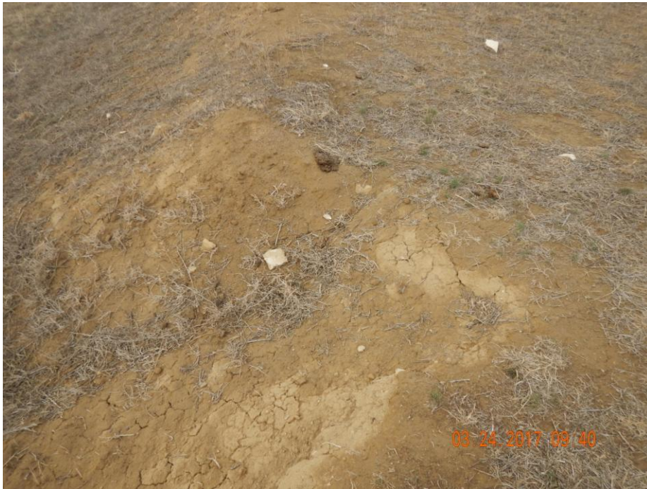
Photo 3: Photo taken from the south end of the location. Photo shows temporary stormwater and sediment control BMPs have not been installed to mitigate stormwater erosion.
