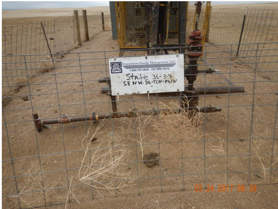
Photo 1: Photo taken from the well head. Inspection doc. #682501708 documented an audible leak occurring from well. Inspector can no longer detect leak. Sign has been placed at well.
