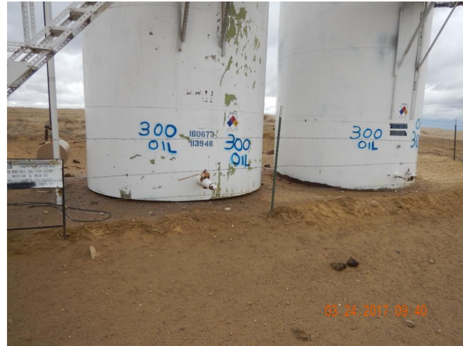
Photo 2: Photo taken from the tank battery. Appropriate labeling has been place. Berm along tank battery still remains in improper function condition.
