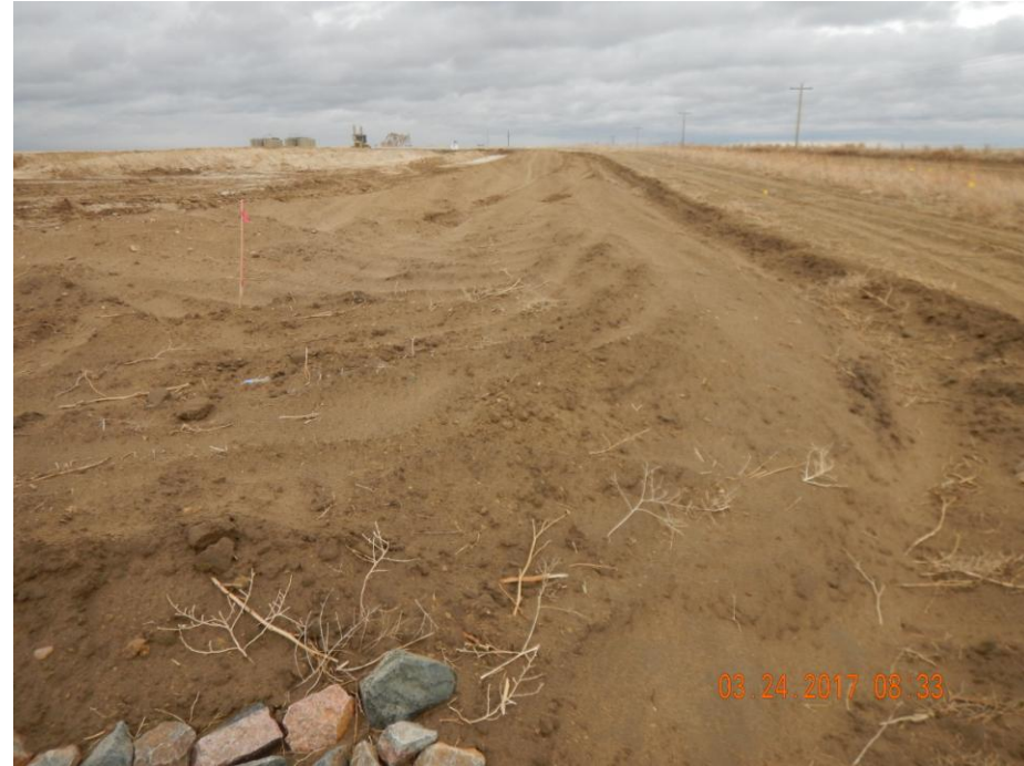
Photo 2: Photo taken from the northwest end of the location facing south. Photo shows stormwater and sediment control ditch along perimeter of the location. Ditch in its current condition is satisfactory as a temporary control for this stage of construction, however, ditch is not consolidated and has been constructed with a steep grade. Alternative BMPs will need to be implemented or ditch will need to be upgraded once pad-construction activities have finished. CDOT recommends ditches be constructed with a grade of 2:1.
