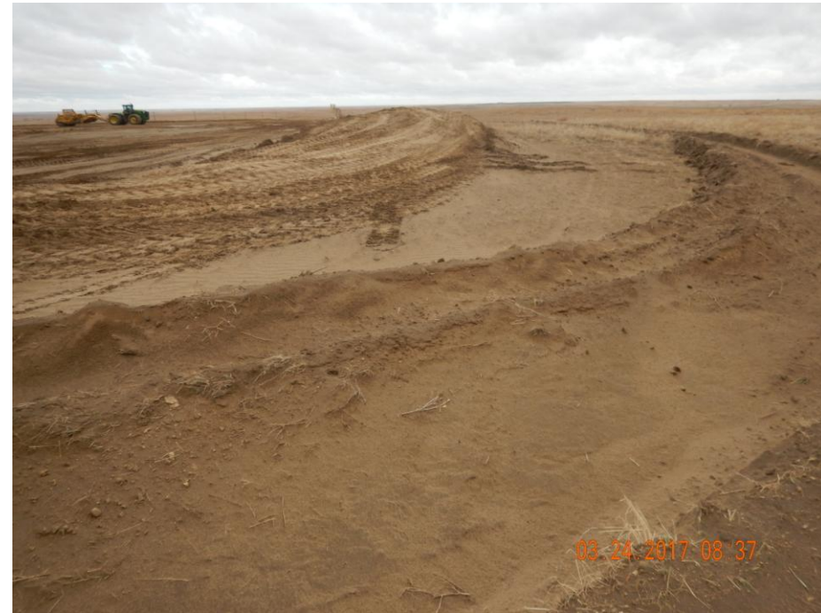
Photo 10: Photo taken from the southeast end of the location facing north. Photo shows stormwater and sediment control ditch along perimeter of the location. Ditch in its current condition is satisfactory as a temporary control for this stage of construction, however, ditch has not been consolidated and has been constructed with a steep grade. Alternative BMPs will need to be implemented or ditch will need to be upgraded once pad-construction activities have finished. CDOT recommends ditches be constructed with a grade of 2:1.
