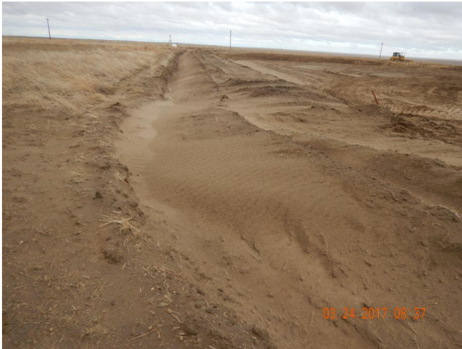
Photo 9: Photo taken from the southeast end of the location facing west. Photo shows stormwater and sediment control ditch appears shallowly constructed, has become inundated with sediment and requires maintenance.
