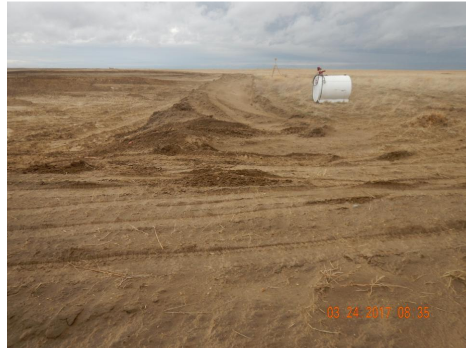
Photo 7: Photo taken from the southwest end of the location facing east. Photo shows stormwater and sediment control ditch along perimeter of the location. Ditch in its current condition is satisfactory as a temporary control for this stage of construction, however, ditch is incomplete in the southwest corner of the location, has not been consolidated and has been constructed with a steep grade. Alternative BMPs will need to be implemented or ditch will need to be upgraded once pad-construction activities have finished. CDOT recommends ditches be constructed with a grade of 2:1.
