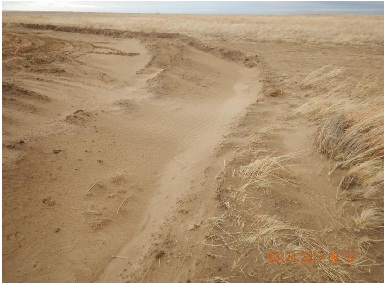
Photo 8: Photo taken from the southeast corner of the location. Photo shows stormwater and sediment control ditch appears shallowly constructed, has become inundated with sediment and requires maintenance.
