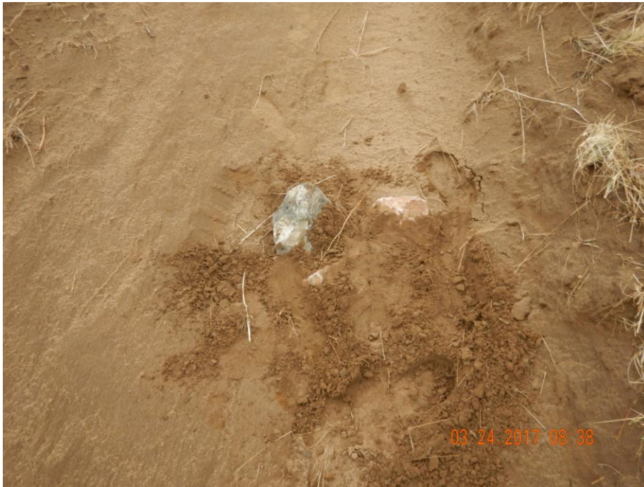
Photo 11: Photo taken from the east end of the location facing southwest. Photo shows rocks in the ditch used as a check-dam. The amount of aggregate and size used is insufficient and inadequate; check-dam has been improperly installed. Check-dam has been inundated with sediment and not in proper functioning condition.
