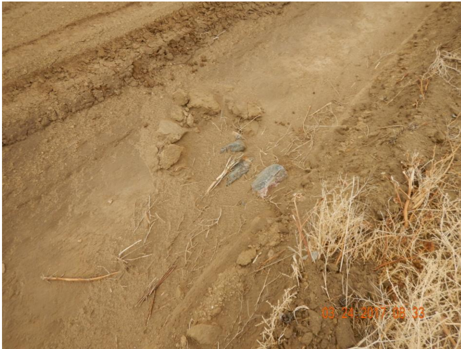
Photo 4: Photo taken from the west end of the location facing southwest. Photo shows rocks in the ditch used as a check-dam. The amount of aggregate and size used is insufficient and inadequate; check-dam has been improperly installed. Check-dam has been inundated with sediment and not in proper functioning condition.
