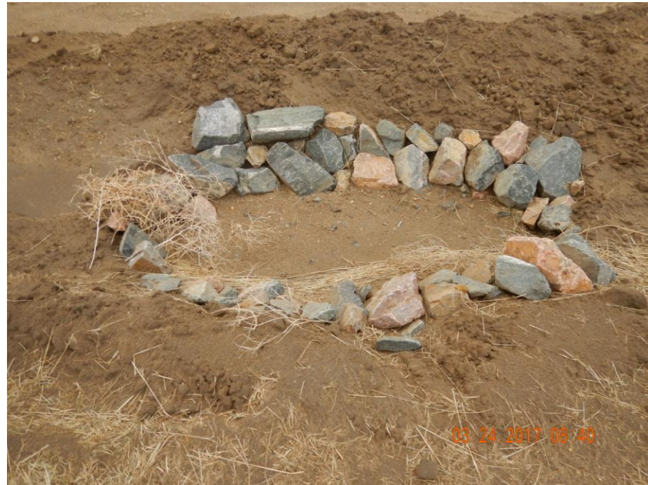
Photo 14: Photo taken from the northeast end of the location. Photo shows sediment trap BMP. BMP has filled with sediment and will require maintenance. The northeast end of the location appears to be the low end topographically. When a large stormwater event occurs, water will likely concentrate in this corner and flow out of the trap/ditch once capacity has been exceeded. Sediment trap does not have an adequate outlet or outlet protection to allow for proper stormwater discharge.
