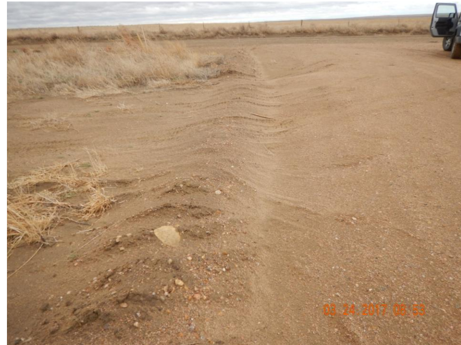
Photo 19: Photo taken from access road north of the location. Photo shows area where access road intersects a second location's access road. Photo shows no vehicle tracking BMPs has been implemented to mitigate sediment tracked from the construction site. In addition, vehicle traffic has traveled over the second access road's ditch BMP; equipment traffic should be kept off BMPs to ensure they function properly. Suggest using an alternative BMP (such as a culvert, cattle guard, ramp, etc...) to mobilize equipment over to mitigate potential negative impacts to stormwater BMPs.
