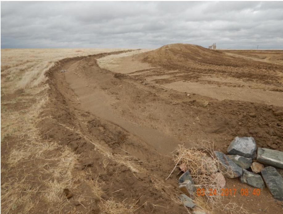
Photo 15: Photo taken from the northeast end of the location facing south. Photo shows stormwater and sediment control ditch along perimeter of the location. Ditch in its current condition is satisfactory as a temporary control for this stage of construction, however, ditch has not been consolidated and has been constructed with a steep grade. Alternative BMPs will need to be implemented or ditch will need to be upgraded once pad-construction activities have finished. CDOT recommends ditches be constructed with a grade of 2:1.
