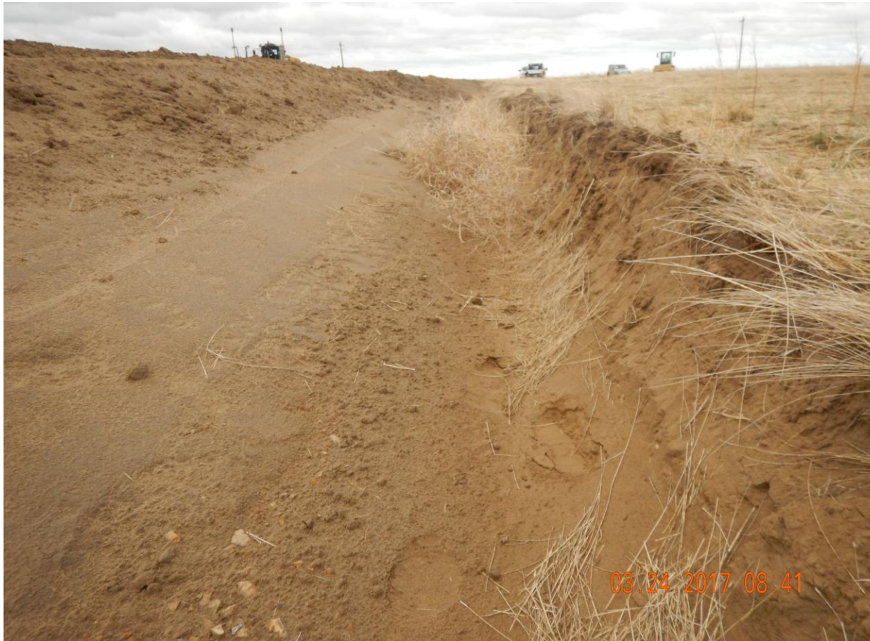
Photo 17: Photo taken from the north end of the location facing west. Photo shows stormwater and sediment control ditch along perimeter of the location. Photo shows ditch has not been consolidated and has been constructed with a steep grade. Alternative BMPs will need to be implemented or ditch will need to be upgraded once pad-construction activities have finished. CDOT recommends ditches be constructed with a grade of 2:1.
