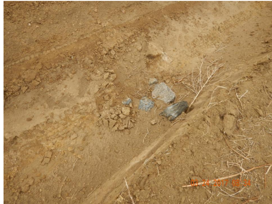
Photo 5: Photo taken from the west end of the location facing southwest. Photo shows rocks in the ditch used as a check-dam. The amount of aggregate and size used is insufficient and inadequate; check-dam has been improperly installed. Check-dam has been inundated with sediment and not in proper functioning condition.
