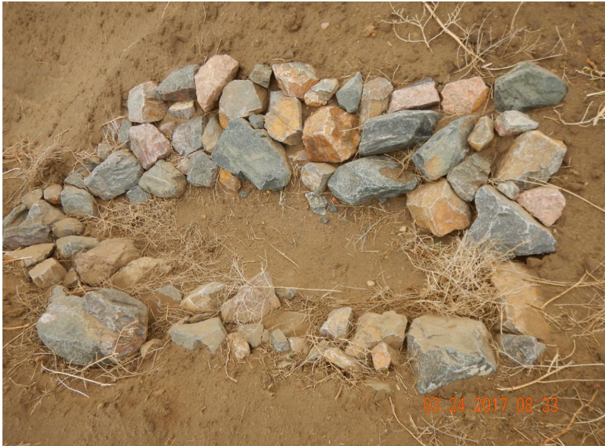
Photo 3: Photo taken from the northwest end of the location. Photo shows sediment trap BMP. BMP has filled with sediment and will require maintenance. It appears only large-sized rock aggregate have been utilized to construct the BMP; using only large aggregates can contribute to erosion degradation as stormwater can be accelerated around or under the material, expanding stormwater impacts and rendering the BMP inadequate.
