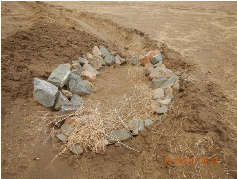
Photo 13: Photo taken from the northeast end of the location. Photo shows sediment trap BMP. BMP has filled with sediment and will require maintenance. The northeast end of the location appears to be the low end topographically. When a large stormwater event occurs, water will likely concentrate in this corner and flow out of the trap/ditch once capacity has been exceeded. Sediment trap does not have an adequate outlet or outlet protection to allow for proper stormwater discharge.
