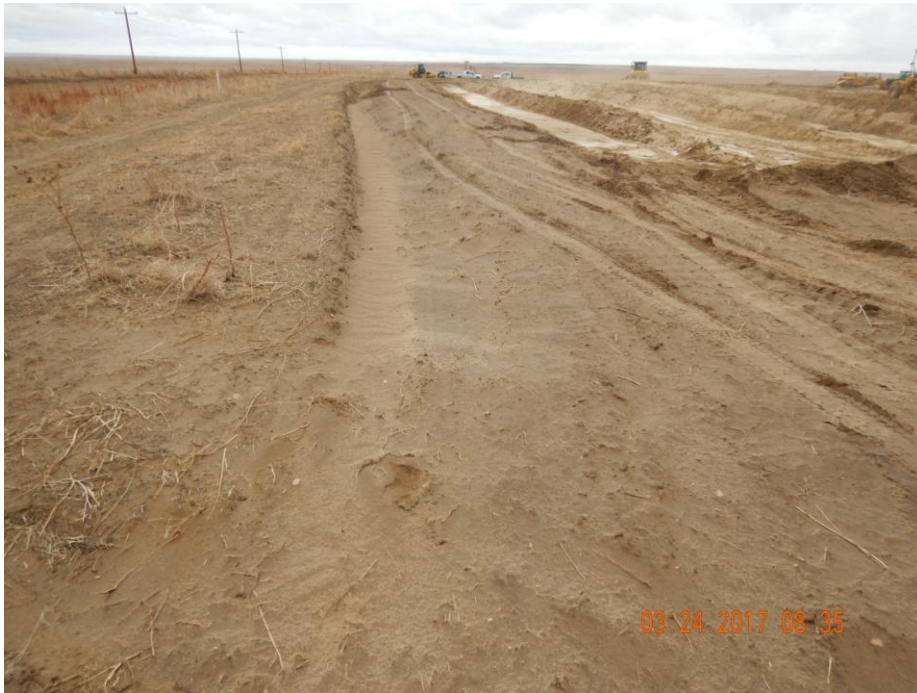
Photo 6: Photo taken from the southwest end of the location facing north. Photo shows stormwater and sediment control ditch along perimeter of the location. Ditch in its current condition is satisfactory as a temporary control for this stage of construction, however, ditch is incomplete in the southwest corner of the location, has not been consolidated and has been constructed with a steep grade. Alternative BMPs will need to be implemented or ditch will need to be upgraded once pad-construction activities have finished. CDOT recommends ditches be constructed with a grade of 2:1.
