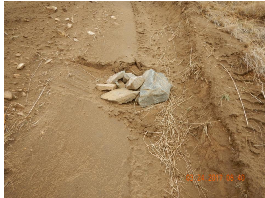
Photo 12: Photo taken from the west end of the location facing southwest. Photo shows rocks in the ditch used as a check-dam. The amount of aggregate and size used is insufficient and inadequate; check-dam has been improperly installed. Check-dam has been inundated with sediment and not in proper functioning condition.
