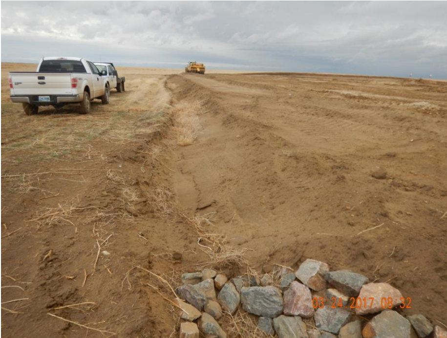
Photo 1: Photo taken from the northwest end of the location facing east. Photo shows stormwater and sediment control ditch along perimeter of the location. Ditch in its current condition is satisfactory as a temporary control for this stage of construction, however, ditch is not consolidated and has been constructed with a steep grade. Alternative BMPs will need to be implemented or ditch will need to be upgraded once pad-construction activities have finished. CDOT recommends ditches be constructed with a grade of 2:1.
