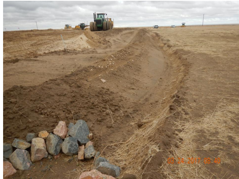
Photo 16: Photo taken from the northeast end of the location facing west. Photo shows stormwater and sediment control ditch along perimeter of the location. Ditch in its current condition is satisfactory as a temporary control for this stage of construction, however, ditch has not been consolidated and has been constructed with a steep grade. Alternative BMPs will need to be implemented or ditch will need to be upgraded once pad-construction activities have finished. CDOT recommends ditches be constructed with a grade of 2:1.
