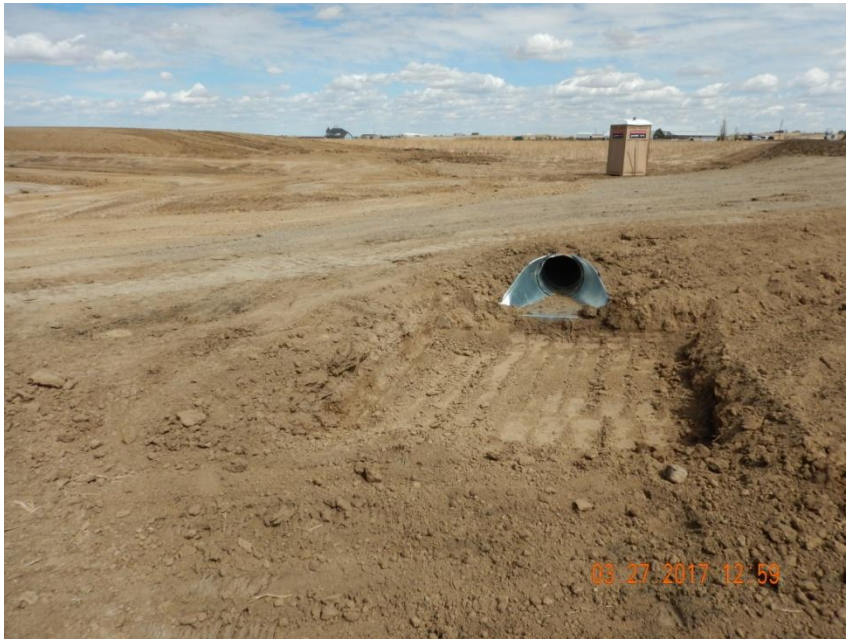
Photo 1. Photo taken from the entrance of location, facing East. Culvert installed for planned diversion ditch.
