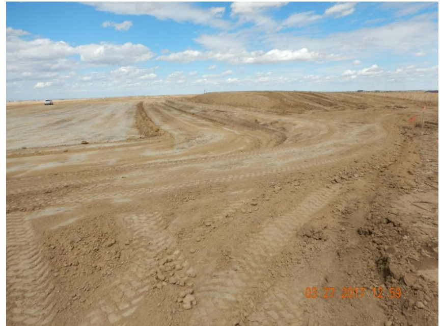
Photo 2. Photo taken from the entrance of location, facing North. Topsoil stockpile stored along the eastern perimeter of the location.
