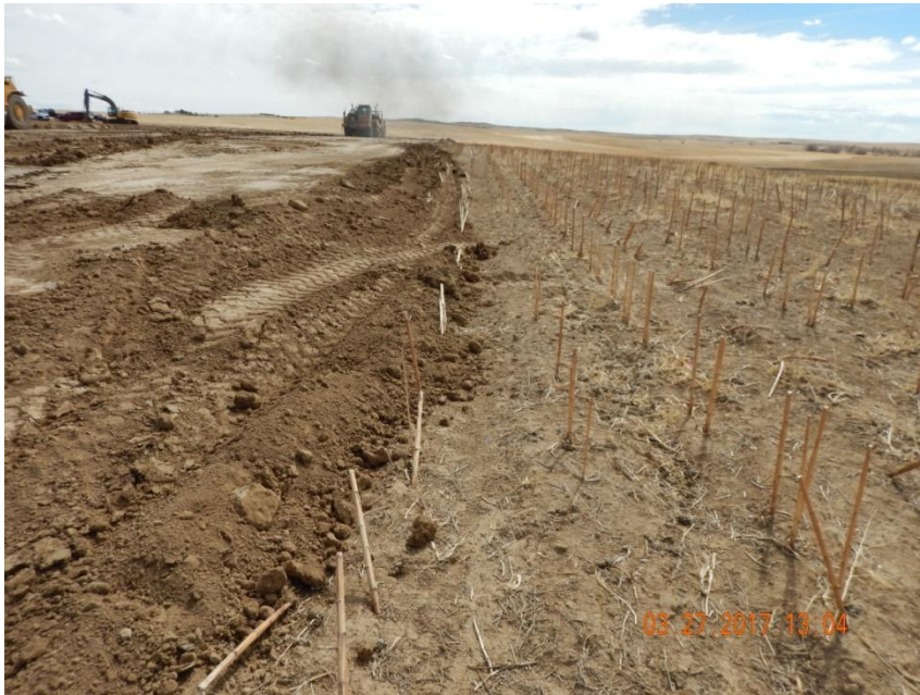
Photo 5. Photo taken from the western location, facing South. No stormwater BMPs have been installed.
