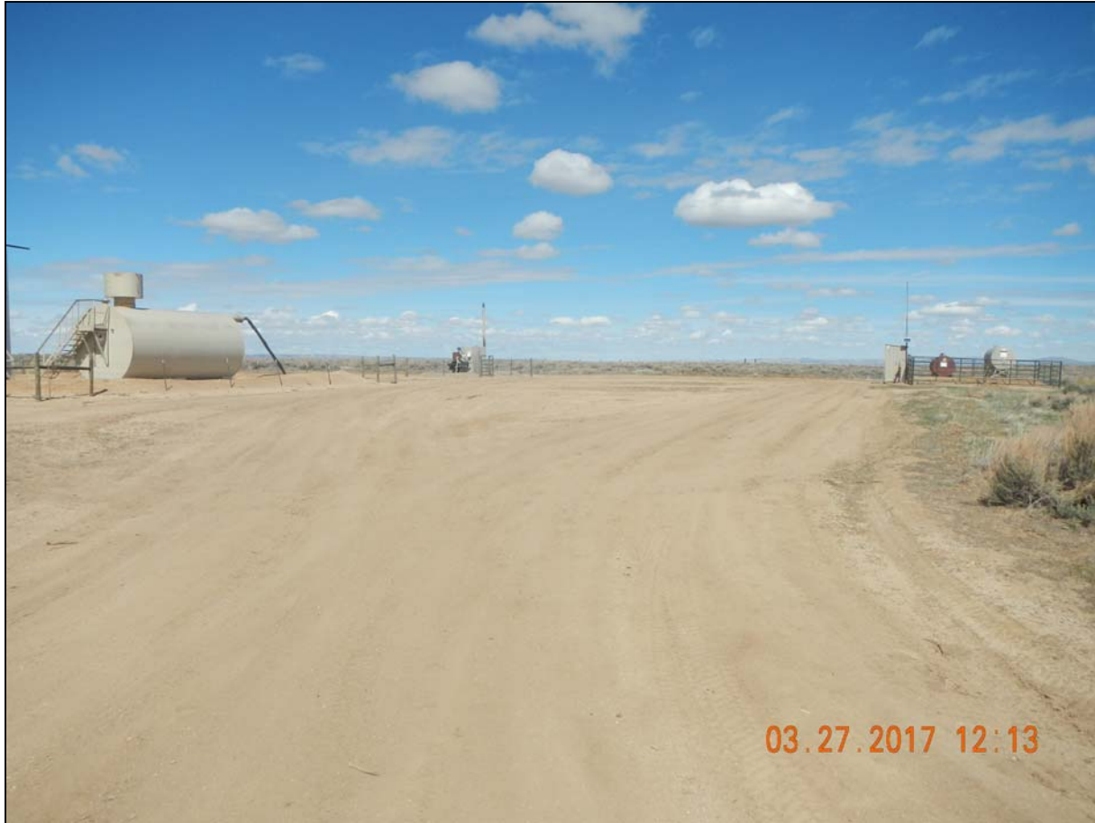
Photo 1. View at entrance to location facing north.
