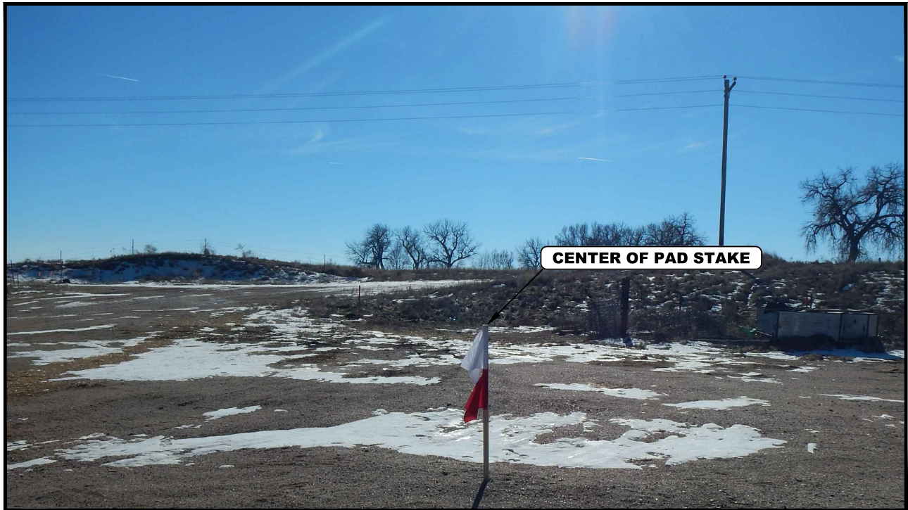
PHOTO: VIEW OF CENTER OF PAD STAKE
