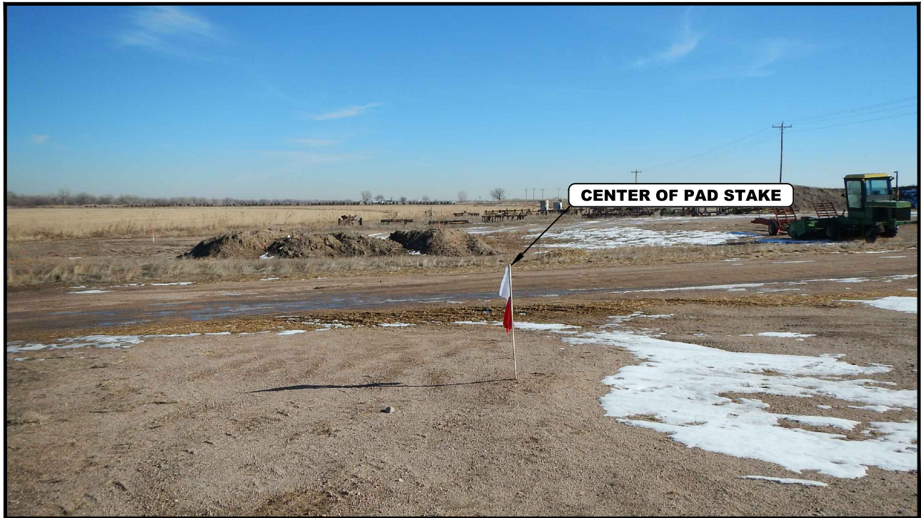
PHOTO: VIEW OF CENTER OF PAD STAKE
