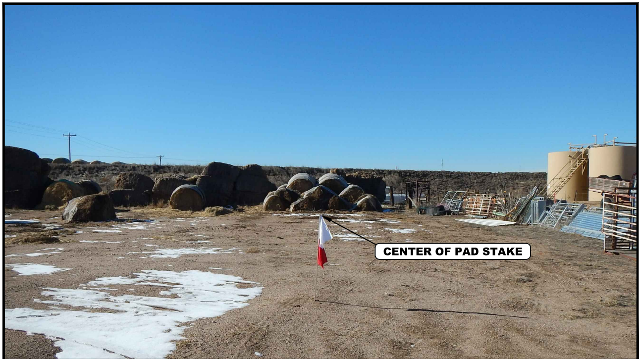
PHOTO: VIEW OF CENTER OF PAD STAKE
