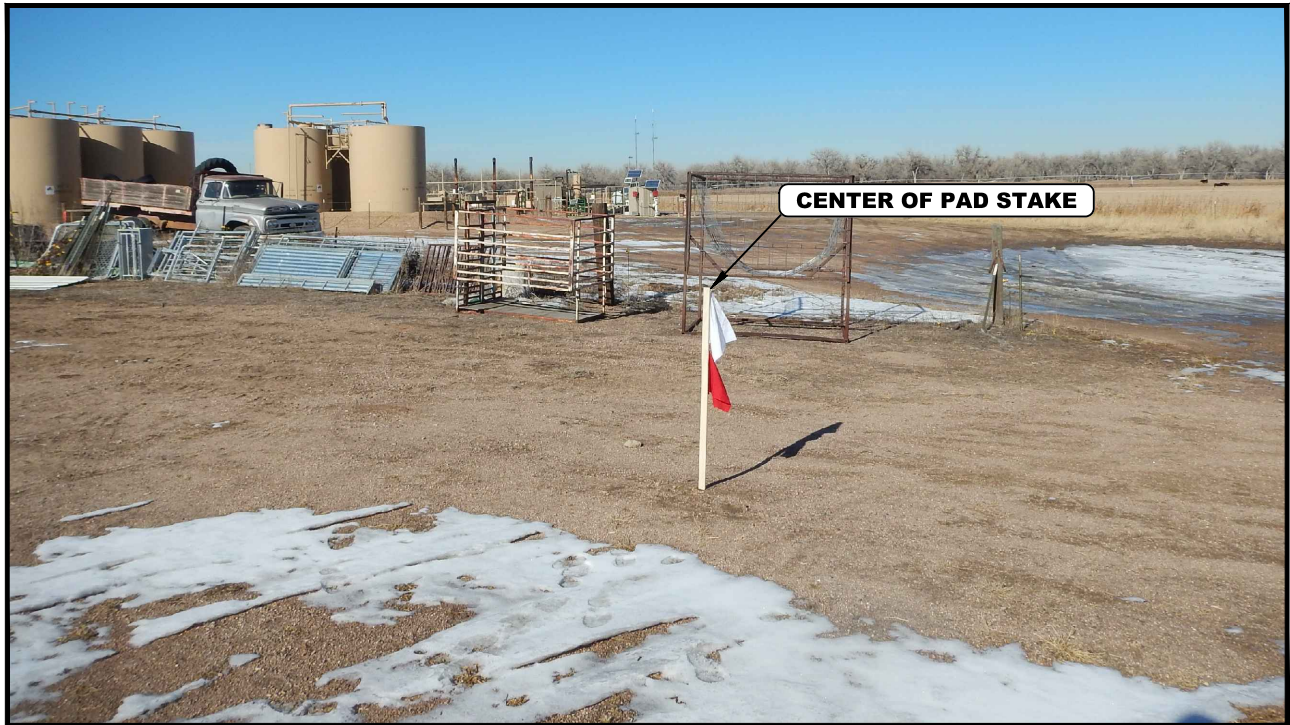
PHOTO: VIEW OF CENTER OF PAD STAKE
