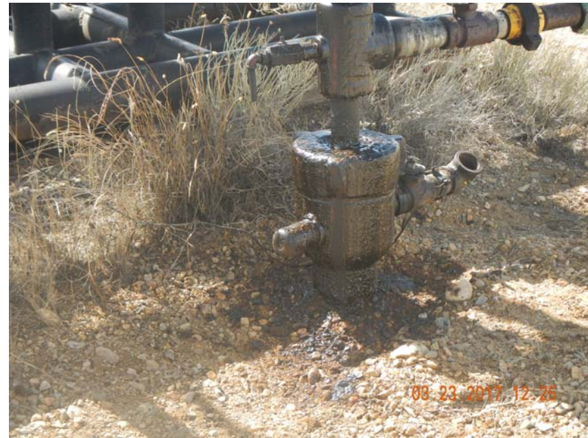
Photo 3. Close-up of leak at wellhead.
