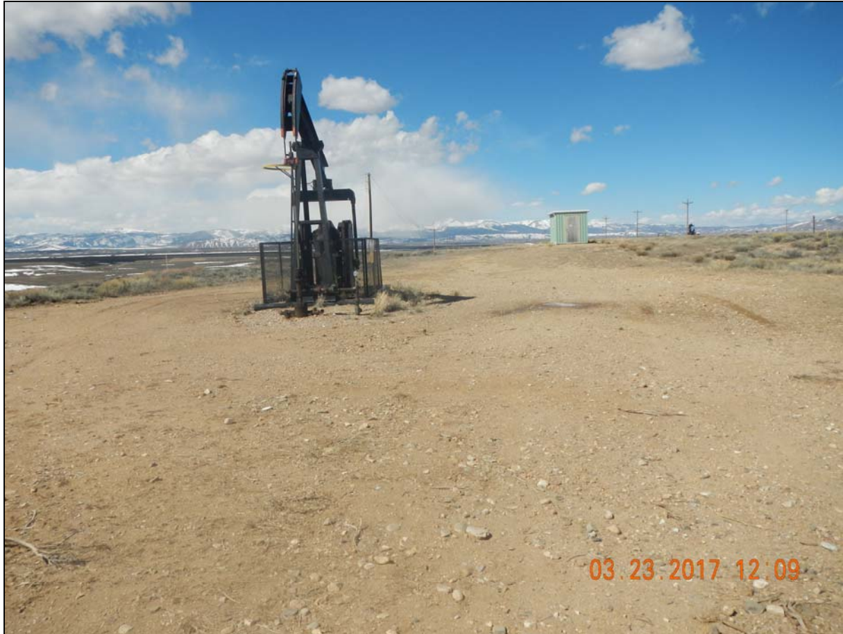
Photo 1. View at entrance to location facing west.
