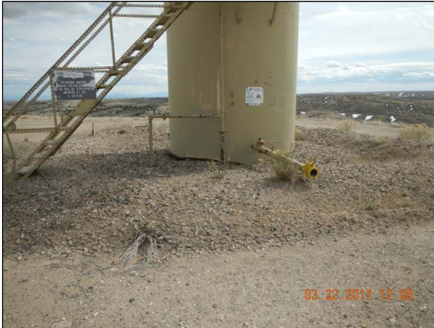
Photo 2. Low berm around crude oil tank.
