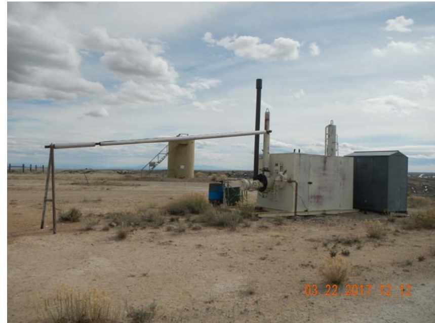
Photo 7. No containment for drums stored next to treater.
