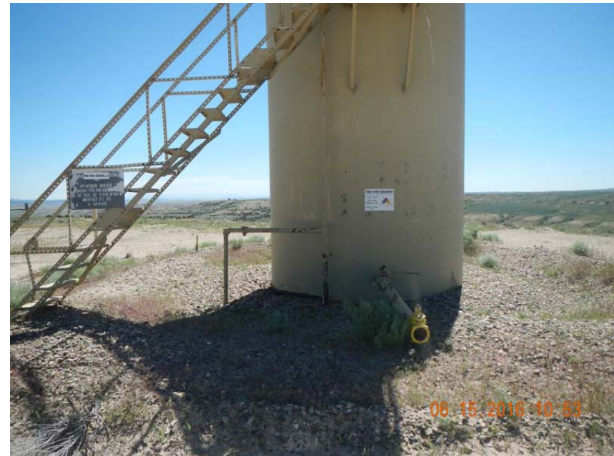
Photo 3. Low berm around crude oil tank during 6/15/2016 inspection.
