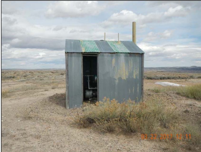
Photo 6. No wildlife protection on exhaust.
