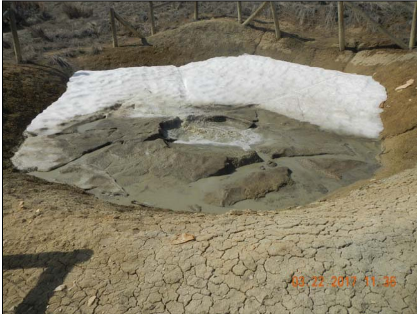
Photo 2. View of pit standing at northeast corner looking southwest. Water in center is bubbling.
