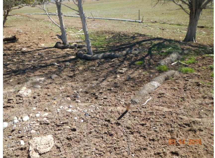
Photo 4: View of wattles that are no longer functioning in the eastern portion of the project area.
