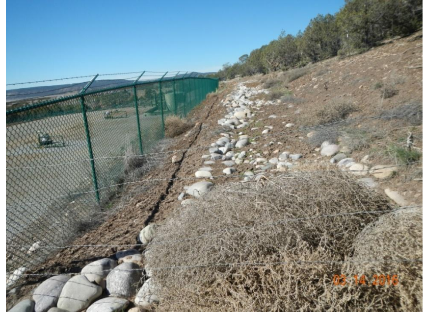
Photo 2: View of the northern portion of the project area from the northeastern corner facing westward. Cobble diversion channel is filling with sediment and will soon need maintenance.
