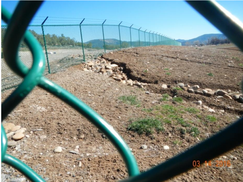
Photo 7: View of an erosional channel forming in the southern portion of the project area that needs stabilization.
