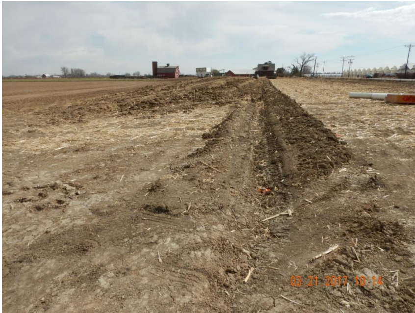
Photo 3. Photo taken from the southwest location, facing East. A ditch and berm BMP has been installed around the perimeter of location. Berm does not appear to be consistently compacted. Topsoil stockpile salvaged and stored along the southern location and along a portion of the southeastern location.
