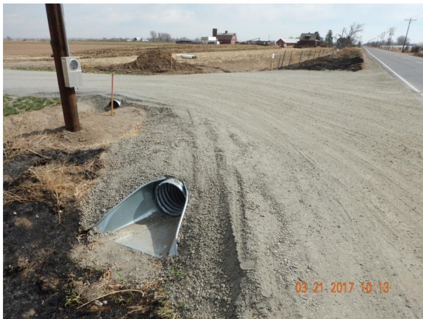
Photo 1. Photo taken from the entrance location, facing East. Two (2) sets of culverts installed in conjunction with existing ditches. Gravel installed at entrance of location.
