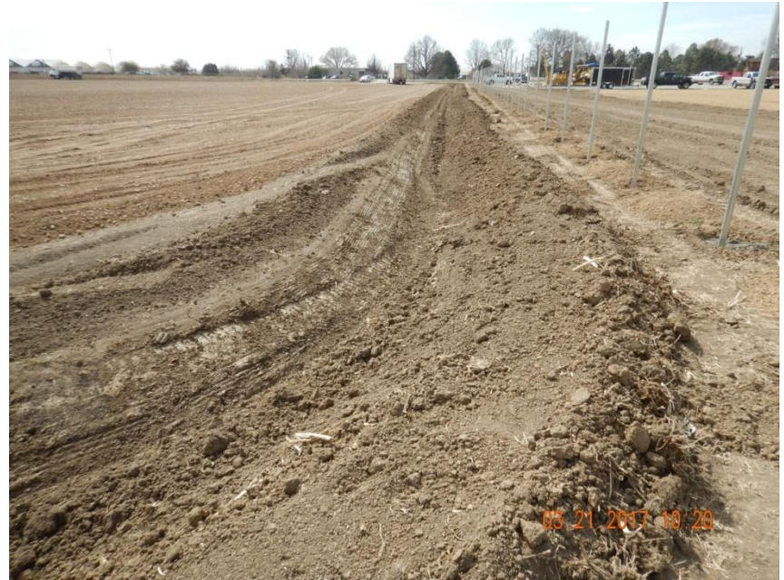
Photo 8. Photo taken from the northwest location, facing South. A ditch and berm BMP has been installed around the perimeter of location. Berm does not appear to be consistently compacted.
