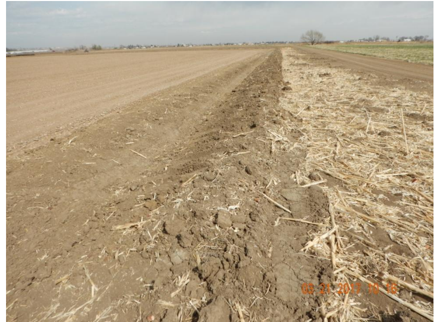
Photo 6. Photo taken from the eastern location, facing North. A ditch and berm BMP has been installed around the perimeter of location. Berm does not appear to be consistently compacted.
