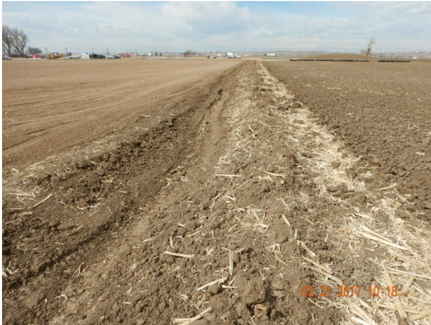
Photo 7. Photo taken from the northern location, facing West. A ditch and berm BMP has been installed around the perimeter of location. Berm does not appear to be consistently compacted.
