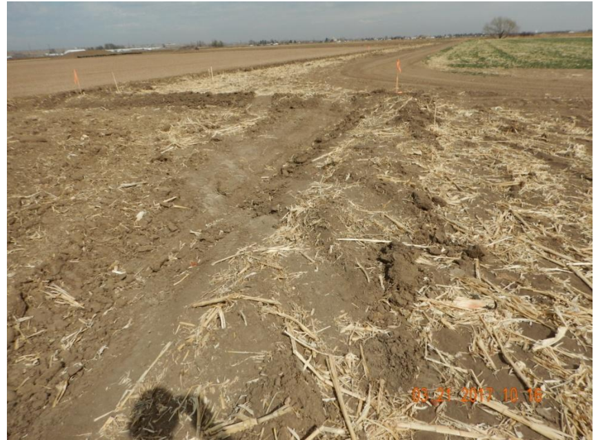
Photo 4. Photo taken from the southeastern location, facing North. A ditch and berm BMP has been installed around the perimeter of location. Berm does not appear to be consistently compacted and vehicle traffic should stay off BMPs to ensure they properly function.
