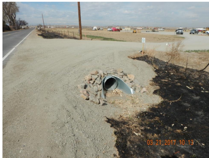
Photo 2. Photo taken from the entrance location, facing West. Two (2) sets of culverts installed in conjunction with existing ditches. Gravel installed at entrance of location.
