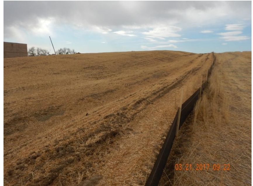
Photo 8. Photo taken from the western location, facing South towards the topsoil stockpile. Topsoil stockpile has been stabilized by crimping straw mulch.
