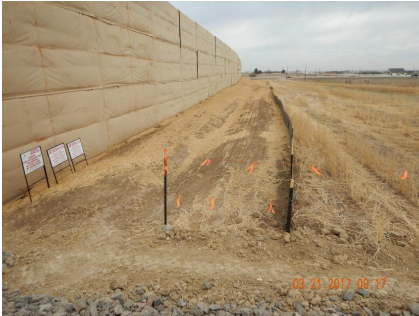
Photo 3. Photo taken from the entrance of location, facing North. A ditch and berm BMP has been installed around the perimeter of the location in conjunction with a silt fence around the perimeter of the location. Also, stormwater areas, cut/fill slopes, and interim areas have been stabilized by crimping straw mulch.
