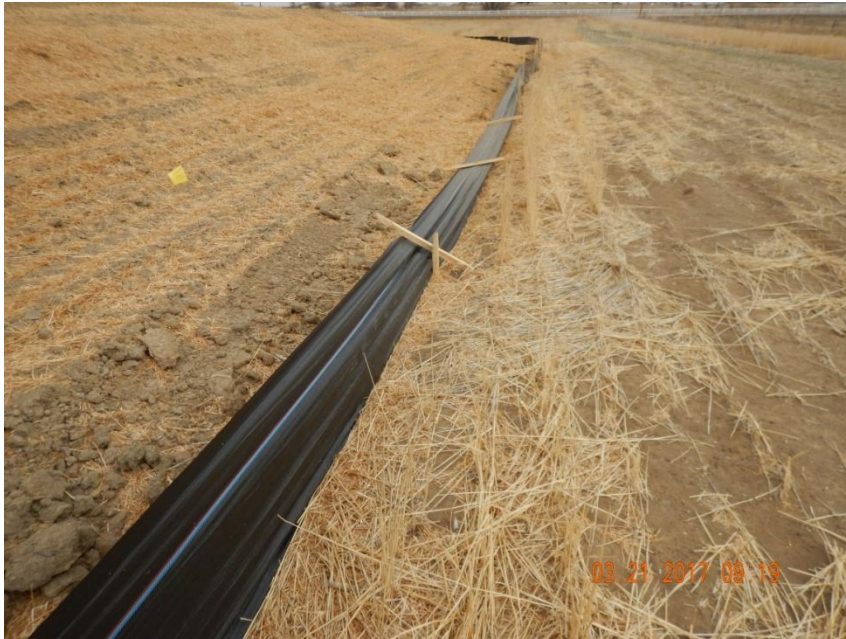
Photo 5. Photo taken from the eastern location, facing North. Silt fence needs repair or maintenance along a portion of the eastern location.
