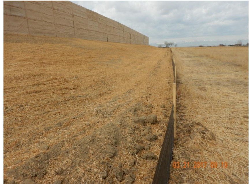
Photo 6. Photo taken from the northeast location, facing West. A ditch and berm BMP has been installed around the perimeter of the location in conjunction with a silt fence around the perimeter of the location. Also, stormwater areas, cut/fill slopes, and interim areas have been stabilized by crimping straw mulch.
