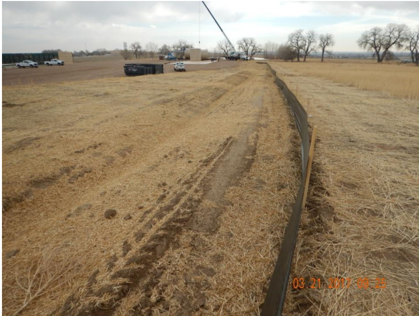
Photo 11. Photo taken from the southwest location, facing East. A ditch and berm BMP has been installed around the perimeter of the location in conjunction with a silt fence around the perimeter of the location. Also, stormwater areas, cut/fill slopes, and interim areas have been stabilized by crimping straw mulch.
