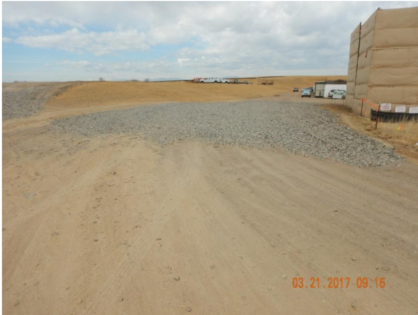
Photo 1. Photo taken from the entrance of location, facing West. Tracking pad installed and appears to be in proper functioning condition. Cut slope along the entrance has been stabilized by crimping straw mulch along the slope.
