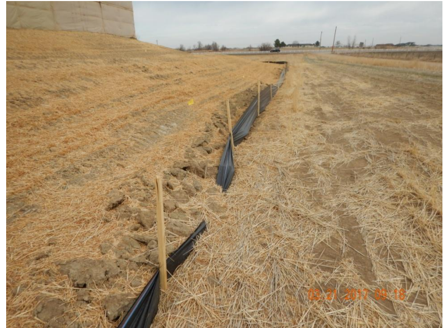
Photo 4. Photo taken from the eastern location, facing North. Silt fence needs repair or maintenance along a portion of the eastern location.
