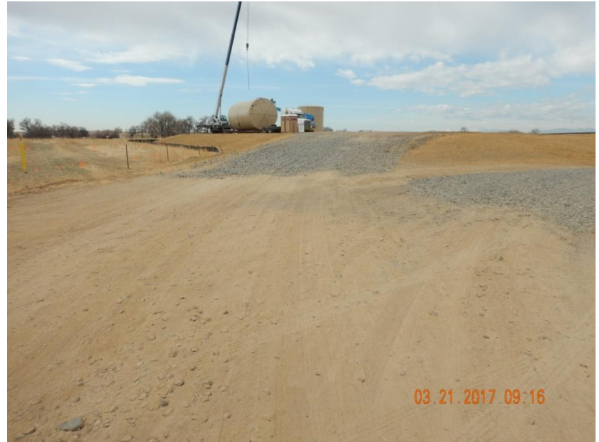
Photo 2. Photo taken from the entrance of location, facing Southwest. Tracking pad installed and appears to be in proper functioning condition.
