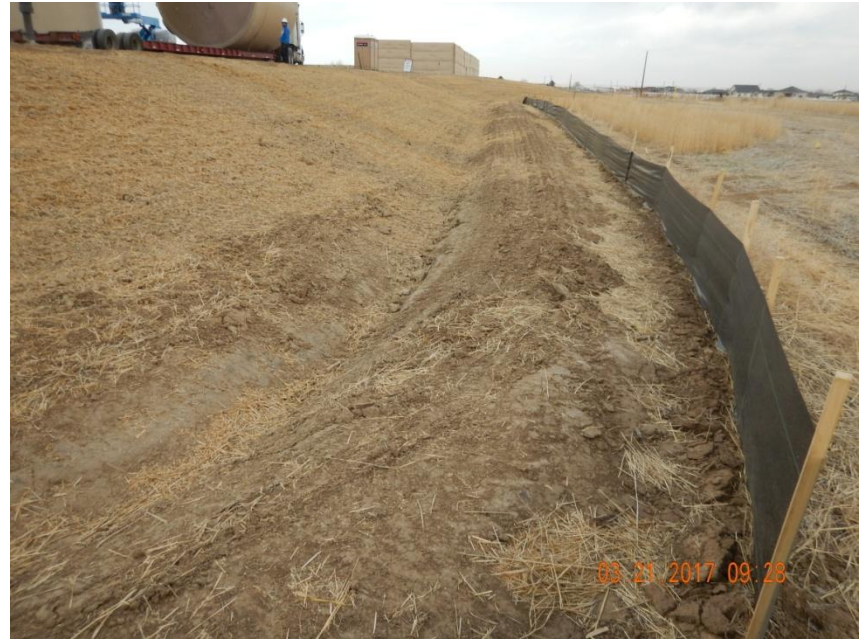
Photo 12. Photo taken from the southeast location, facing North. A ditch and berm BMP has been installed around the perimeter of the location in conjunction with a silt fence around the perimeter of the location. Also, stormwater areas, cut/fill slopes, and interim areas have been stabilized by crimping straw mulch.
