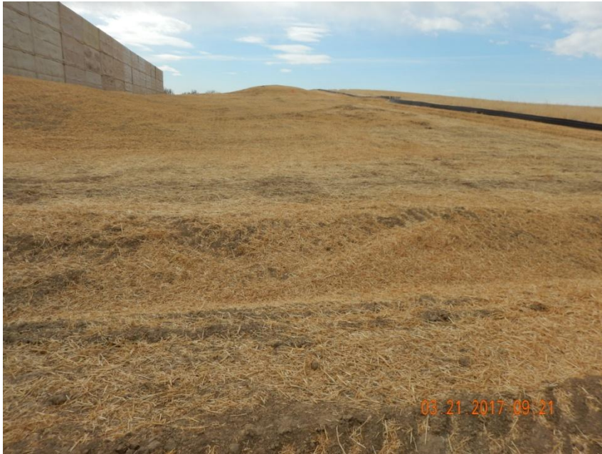
Photo 7. Photo taken from the northwest location, facing South. A ditch and berm BMP has been installed around the perimeter of the location in conjunction with a silt fence around the perimeter of the location. Also, stormwater areas, cut/fill slopes, and interim areas have been stabilized by crimping straw mulch.
