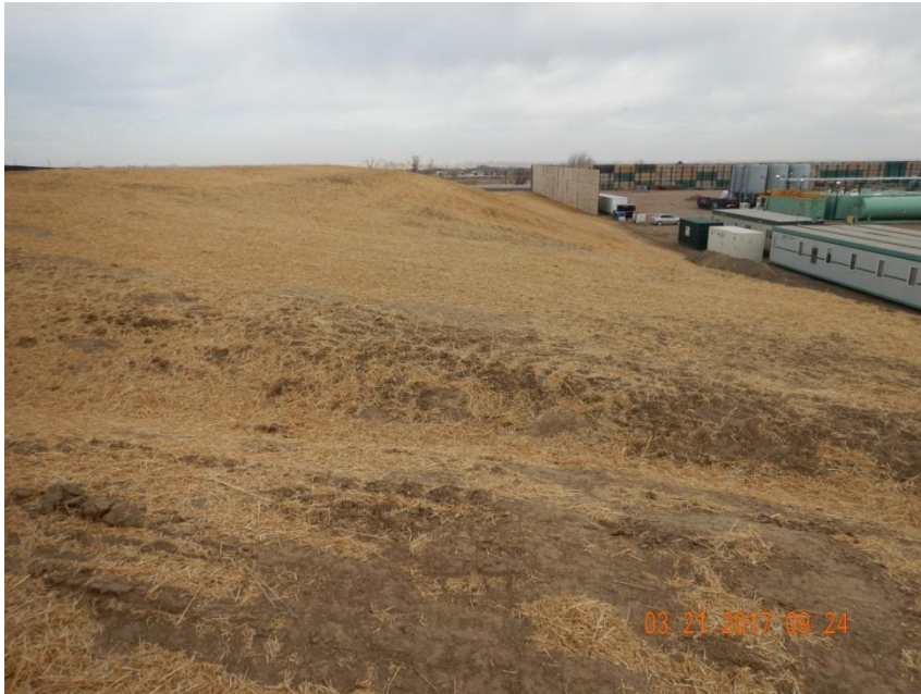
Photo 9. Photo taken from the southwest location, facing North. A ditch and berm BMP has been installed around the perimeter of the location in conjunction with a silt fence around the perimeter of the location. Also, stormwater areas, cut/fill slopes, and interim areas have been stabilized by crimping straw mulch.
