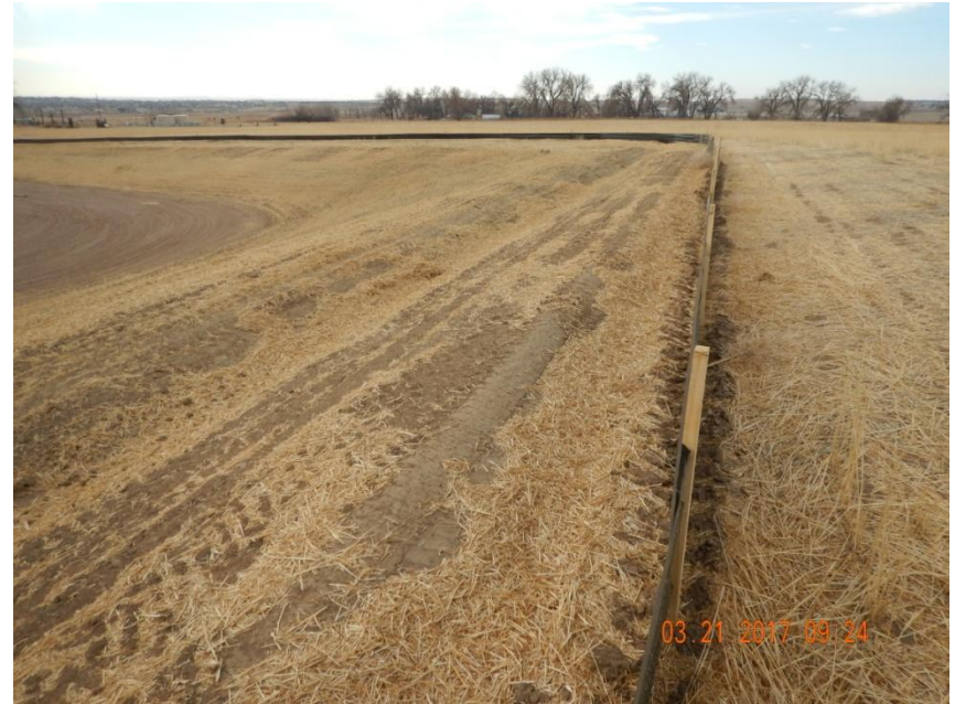
Photo 10. Photo taken from the southwestern location, facing South. A ditch and berm BMP has been installed around the perimeter of the location in conjunction with a silt fence around the perimeter of the location. Also, stormwater areas, cut/fill slopes, and interim areas have been stabilized by crimping straw mulch.
