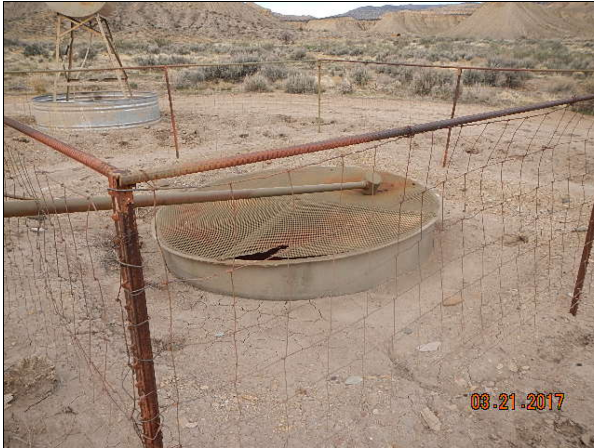
Photo 1. Tank has no signage and bird protection is damaged.
