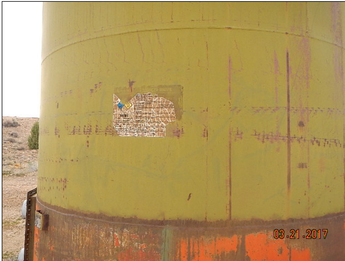
Photo 1. NFPA label is faded. No capacity or emergency contact info on tank.
