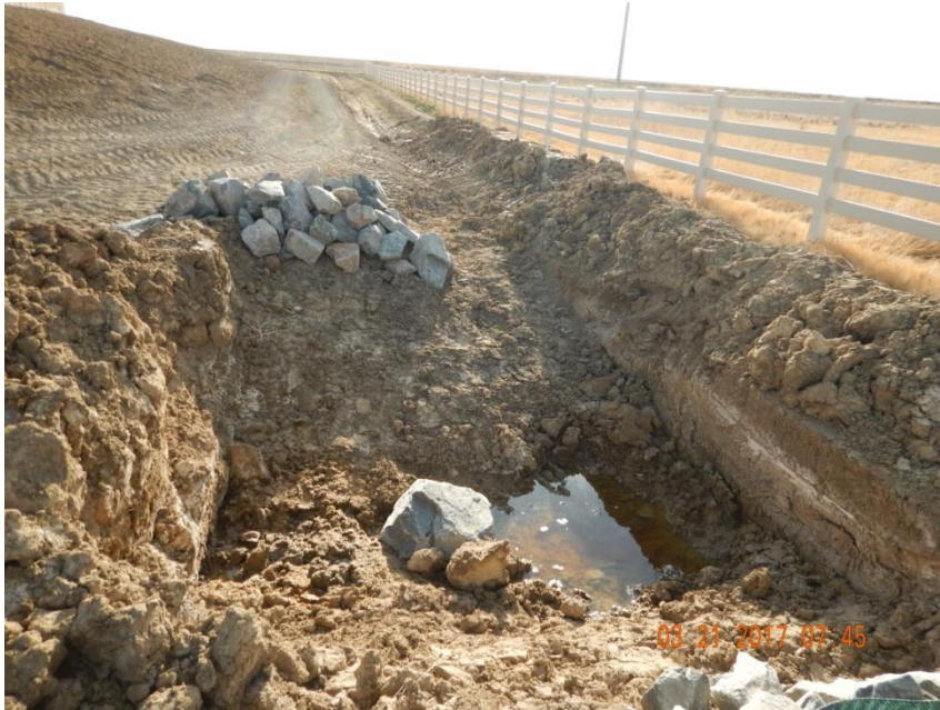
Photo 1. Photo taken from the southwest sediment trap, facing East. Ground water encountered while constructing the sediment trap. Rip rap installed for both inlet and outlet protection has not been installed properly. Unconsolidated soil material dug out from the sediment trap has not been properly compacted.
