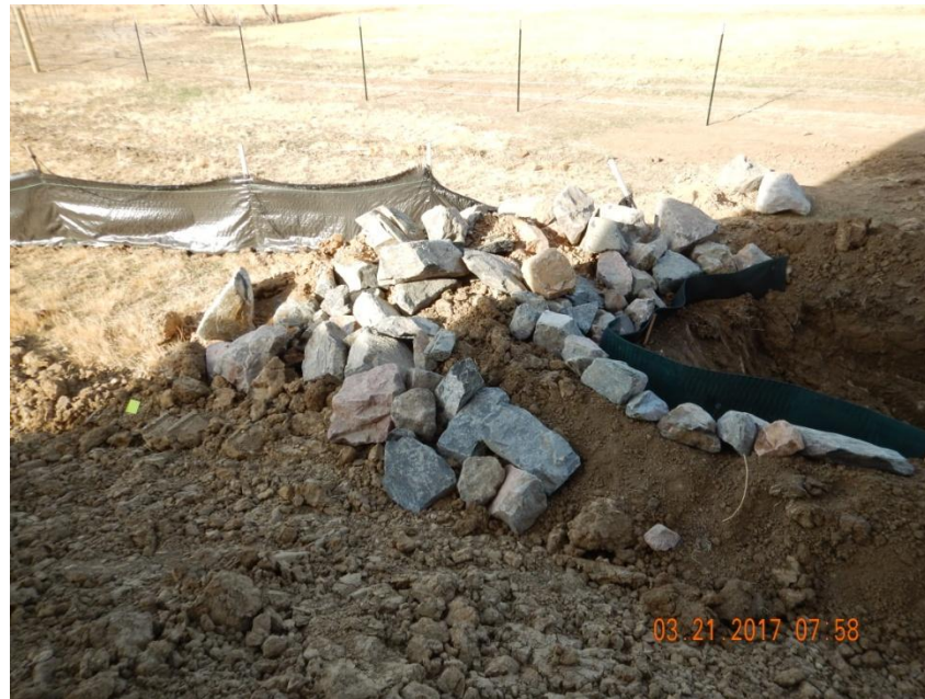
Photo 7. Photo taken of the outlet protection on the western sediment trap, facing West. Rip rap does not appear to be properly installed to function as outlet protection. Rip rap material has fallen onto the S-fence BMP which may likely diminish to S-fence BMP.
