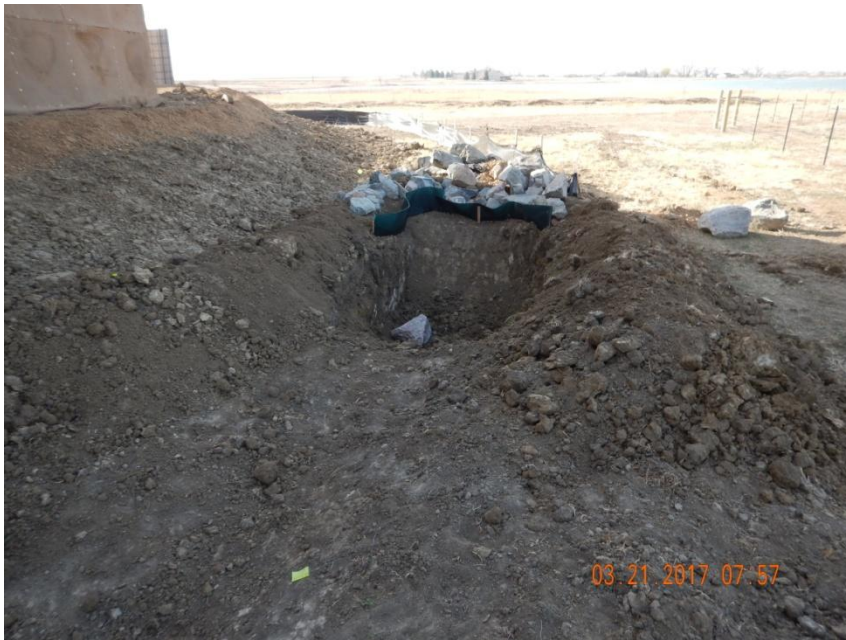
Photo 5. Photo taken from the western sediment trap, facing South. Unconsolidated soil material dug out from the sediment trap has not been properly compacted.
