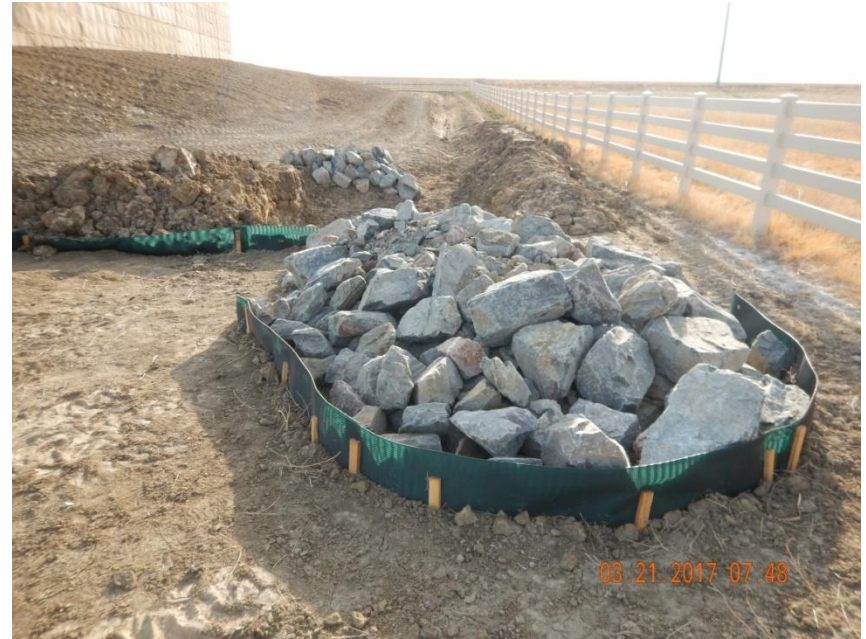
Photo 2. Photo taken from the southwest sediment trap, facing East. Appears this is supposed to serve as outlet protection but it does not connect with the outfall area of the sediment trap. Appears the rip rap was dumped at location without properly installing the BMP to even be a functioning part of the sediment trap.
