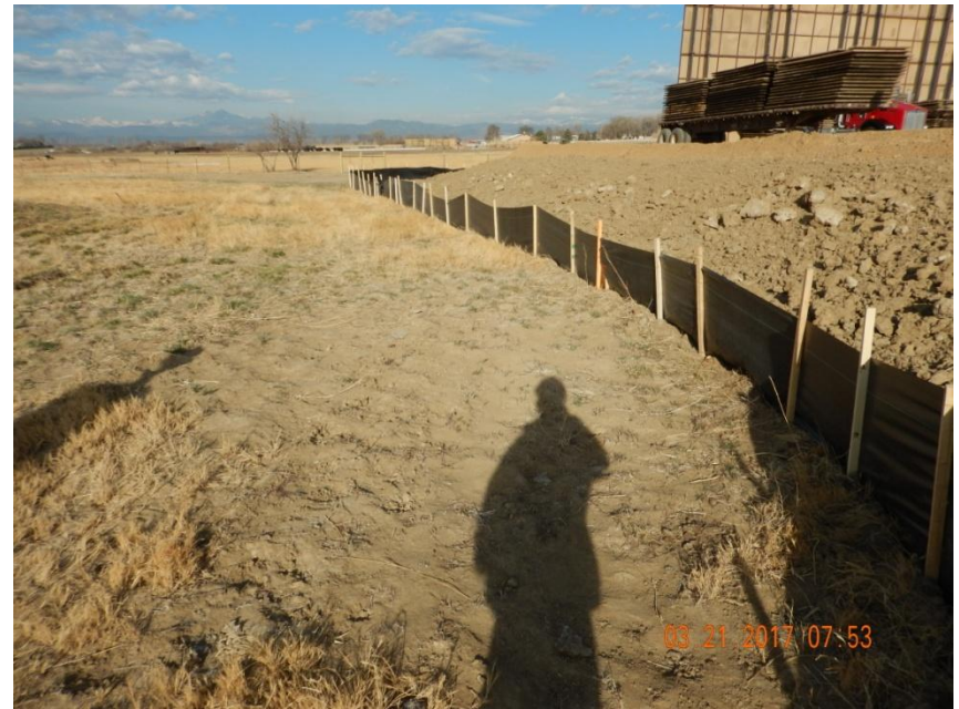
Photo 4. Photo taken from the southwestern location, facing West. Silt fence BMP has been repaired and appears to be in proper functioning condition.
