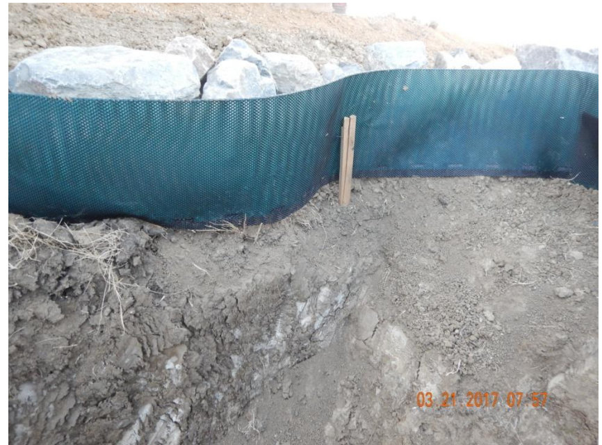
Photo 6. Photo taken of the S-fence BMP along the sediment trap which has not been properly trenched or installed.
