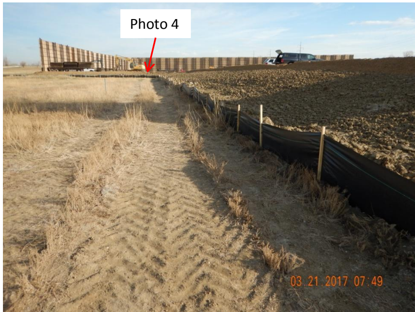
Photo 3. Photo taken from the southwest location, facing North. Silt fence BMP has been repaired and appears to be in proper functioning condition.
