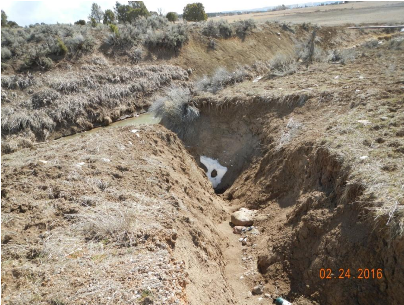
Photo 6: View of erosional channel approximately three feet wide and deep in the southern portion of the project area, flowing into an irrigation canal.
