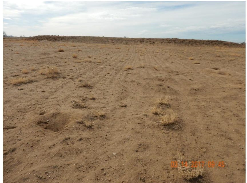
Photo 14. Photo taken from the northwest area, facing South. Approximately 4.0 acres have been disturbed but the area has not been compacted, covered, paved, or otherwise stabilized to minimize dust and erosion.
