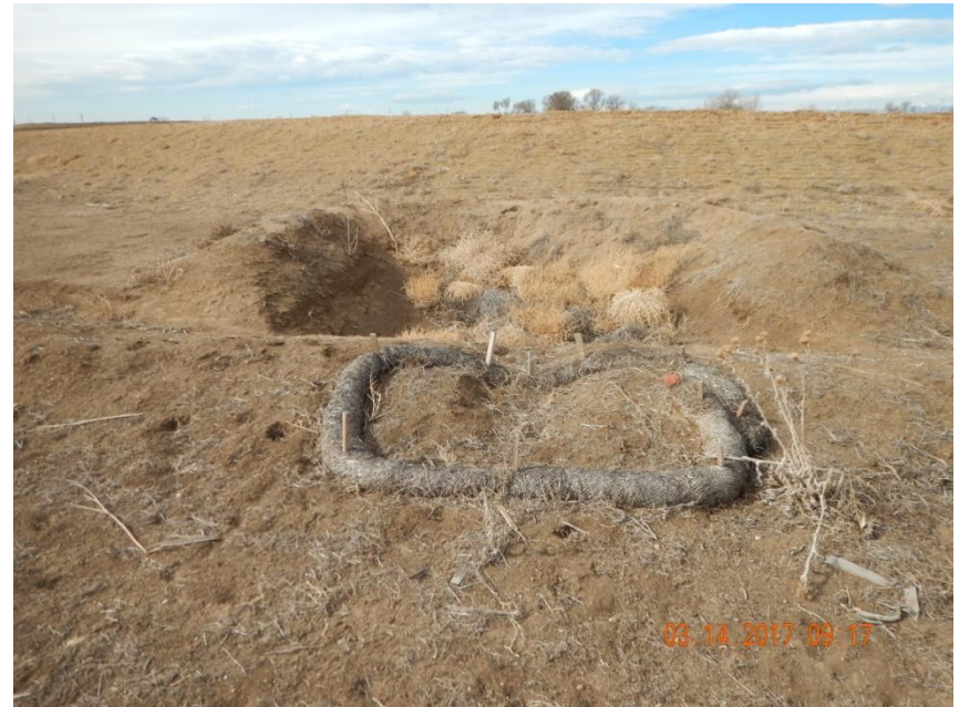
Photo 6. Photo taken from the northeast sediment trap, facing Southwest. Outlet protection in the form of straw wattles may need maintenance or repair.
