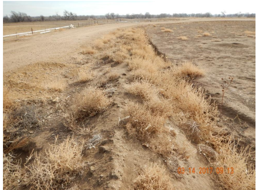
Photo 4. Photo taken from the northwestern location, facing East. A ditch and berm BMP has been installed around the perimeter of the location. Russian thistle found throughout ditch and berm BMP, acting as debris.
