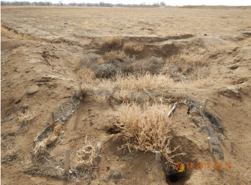
Photo 3. Photo taken from the northwest sediment trap, facing Southeast. Outlet protection in the form of straw wattles need to be repaired.
