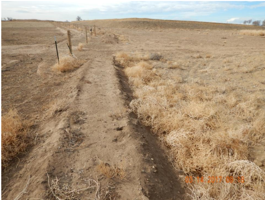
Photo 7. Photo taken along the eastern location, facing South. A ditch and berm BMP has been installed around the perimeter of the location. Russian thistle found throughout ditch and berm BMP, acting as debris. Russian thistle accumulating in ditches.
