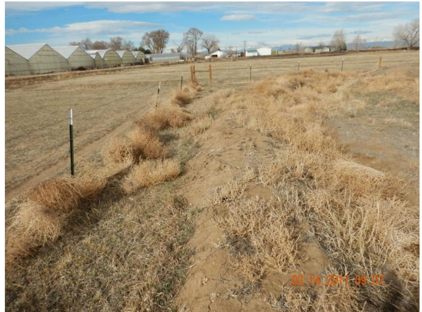
Photo 2. Photo taken from the southwest location, facing West. A ditch and berm BMP has been installed around the perimeter of the location. Russian thistle found throughout ditch and berm BMP, acting as debris. Russian thistle accumulating in ditches and perimeter fence.
