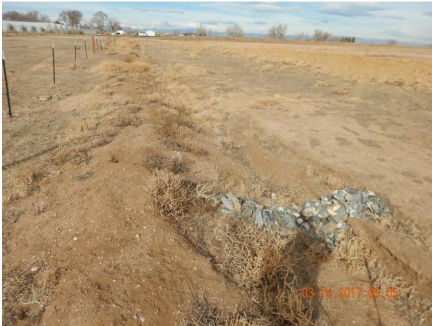
Photo 1. Photo taken from the southern location, facing West. A ditch and berm BMP has been installed around the perimeter of the location. Russian thistle found throughout ditch and berm BMP, acting as debris. Russian thistle accumulating in ditches.
