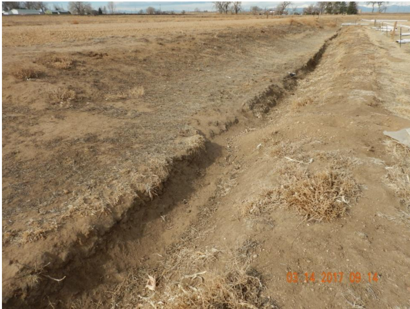
Photo 5. Photo taken from the northeastern location, facing West. A ditch and berm BMP has been installed around the perimeter of the location. Prairie dogs have established throughout the location, sometimes along the BMPs where maintenance is needed.
