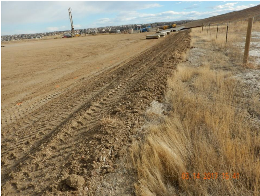
Photo 5. Photo taken from the western location, facing South. The east-facing cut slope appears to be stabilized.
