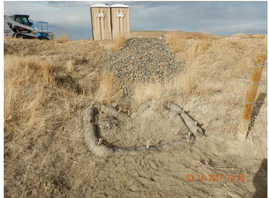
Photo 10. Photo taken just northeast of previous location, facing North. Sediment trap installed with outlet protection in the form of straw wattles. Straw wattles appear to need maintenance or repairs.
