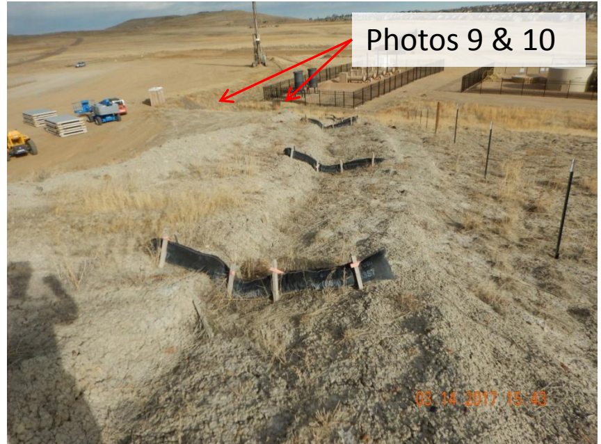
Photo 8. Photo taken from the southwestern location along the uphill side of the cut slope, facing East. Wattles have been installed in conjunction with the ditch BMP.
