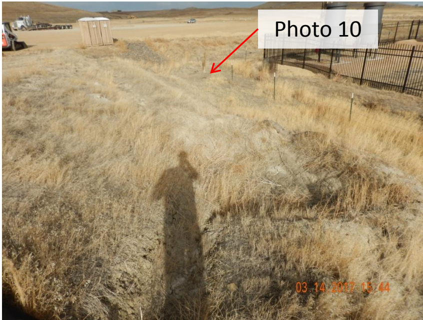
Photo 9. Photo taken from the downhill side of the cut slope, facing East. Vegetative growth makes it difficult to observe but outlet protection in the form of straw wattles may need maintenance or repair.
