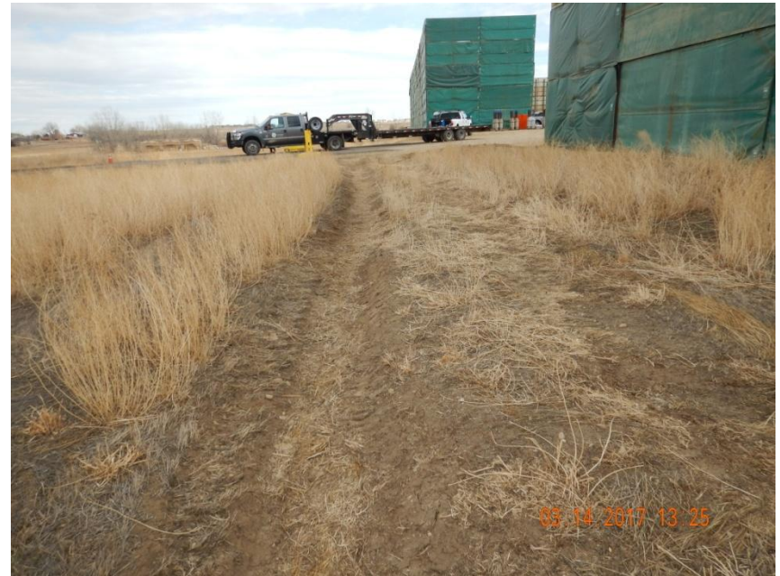
Photo 12. Photo taken from the entrance of the well site, facing East. A ditch and berm BMP has been installed around the perimeter of the location.
