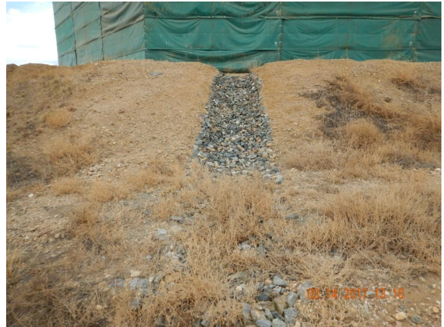
Photo 4. Photo taken from the northeastern location, facing South. The northeast fill slope has a stabilized outlet that is directed to the ditch and berm BMP.
