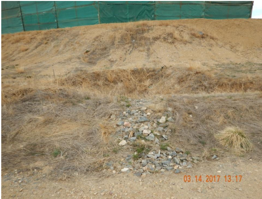
Photo 5. Photo taken from the northeast sediment trap, facing Southwest. Stabilized outlet in the form of rip rap has been installed.
