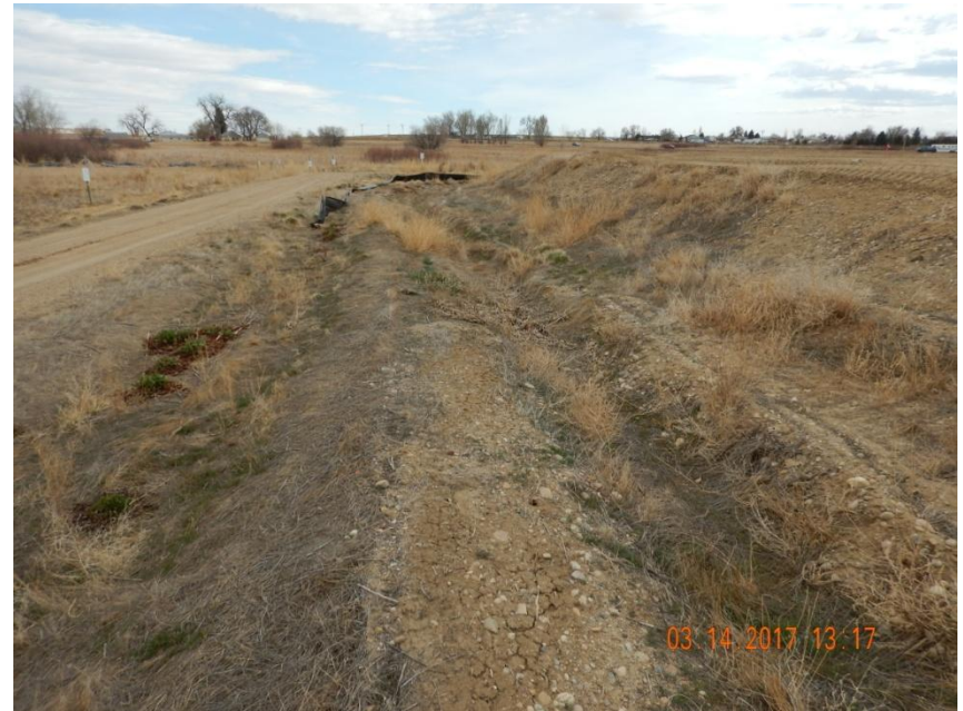
Photo 6. Photo taken from the northeastern location, facing South. A ditch and berm BMP has been installed around the perimeter of the location. Canada thistle vegetative growth from last year was observed throughout the eastern location.
