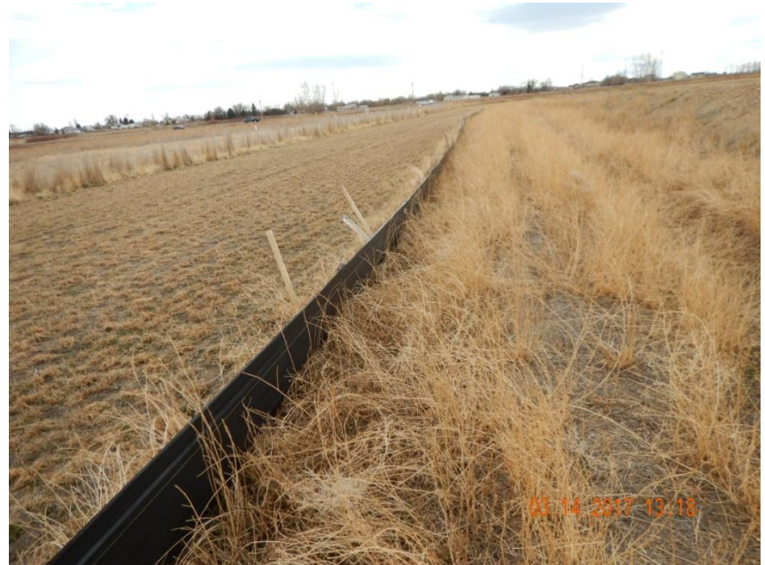
Photo 8. Photo taken from the eastern location, facing South. A ditch and berm BMP has been installed around the perimeter of the location in conjunction with silt fence. Silt fence is in disrepair and needs maintenance.
