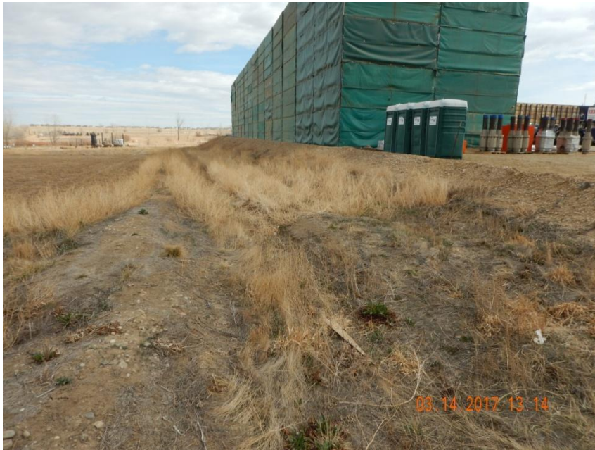
Photo 3. Photo taken from the entrance of the well site, facing East. Vegetative growth makes it difficult to observe but a ditch and berm BMP has been installed around the perimeter of the location.
