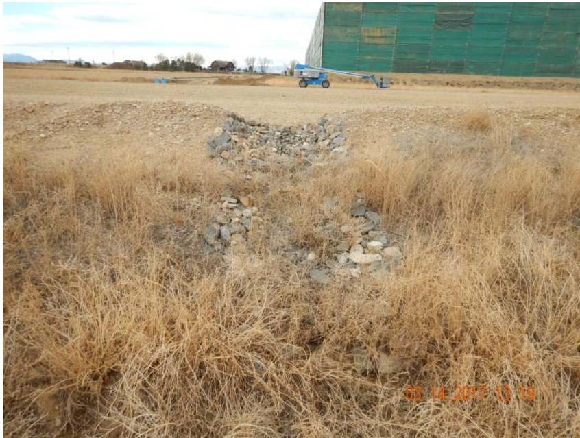
Photo 9. Photo taken from the eastern location, facing West. Fill slope has a stabilized outlet that is directed to the ditch and berm BMP.
