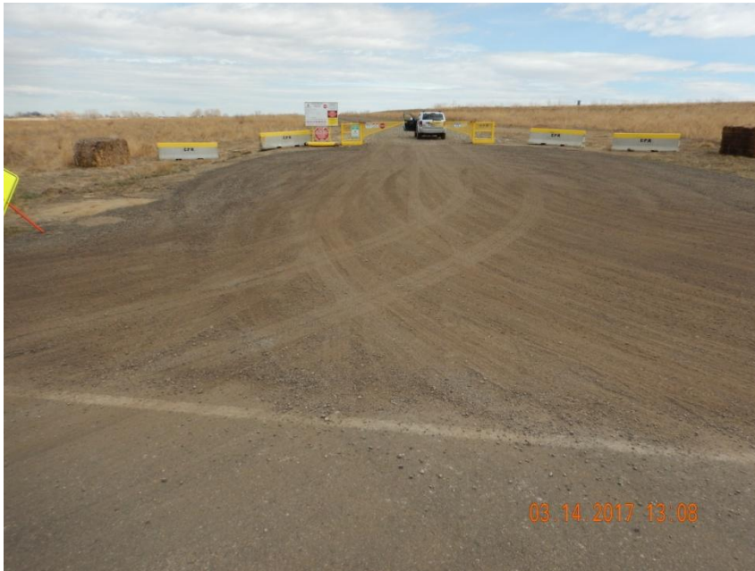
Photo 1. Photo taken from the entrance of location off County Road 3 1/4, facing East. Vehicle tracking pad installed.
