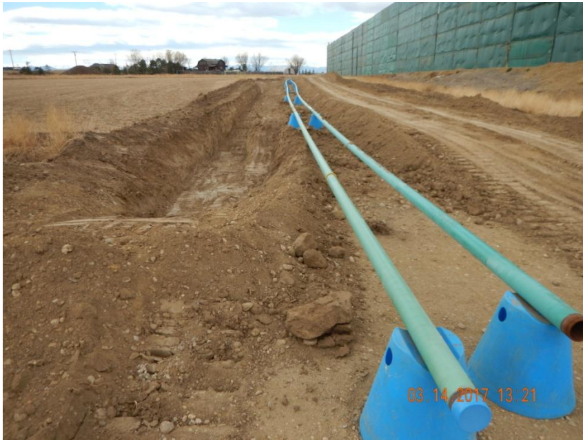
Photo 11. Photo taken from the southern location, facing West. Pipeline construction occurring during inspection. A ditch and berm BMP appeared to be installed around the southern of the location but may need additional maintenance from pipeline construction disturbance.
