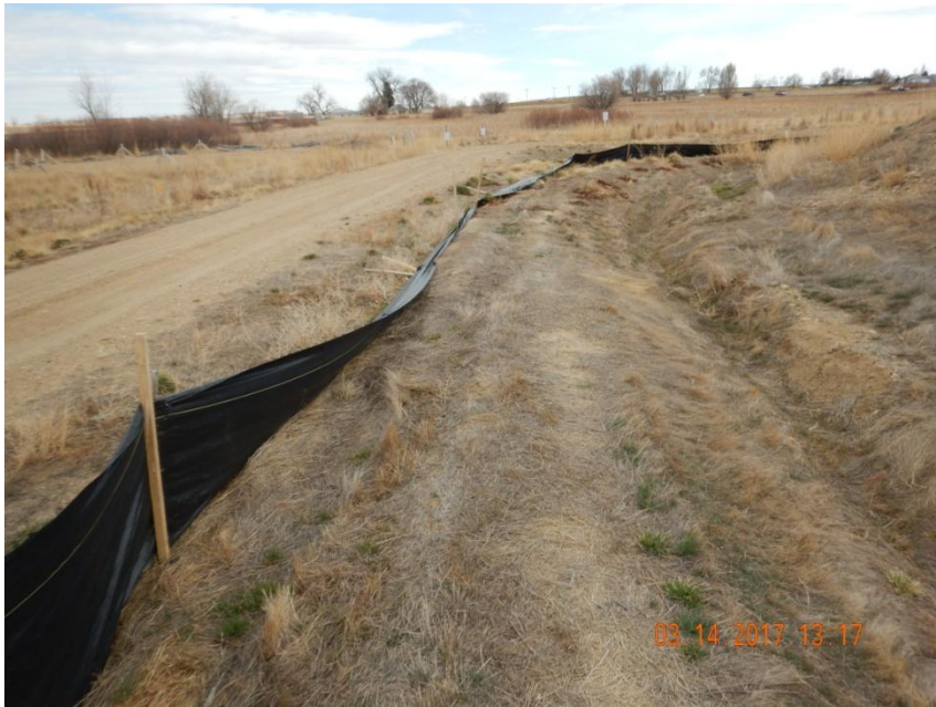
Photo 7. Photo taken from the eastern location, facing South. A ditch and berm BMP has been installed around the perimeter of the location in conjunction with silt fence. Silt fence is in disrepair and needs maintenance. Canada thistle vegetative growth from last year was observed throughout the eastern location.
