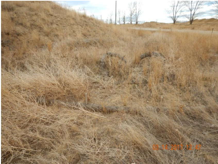
Photo 13. Photo taken from the northwest sediment trap, facing South. Vegetative growth makes it difficult to observe but outlet protection in the form of straw wattles may need maintenance or repair. Some sediment discharge was observed outside of the outlet protection (i.e. wattle). Wattles do not appear to be properly installed (trenched and backfilled).
