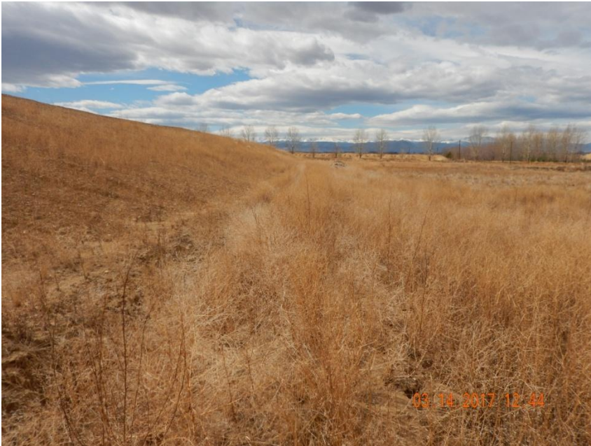
Photo 11. Photo taken from the northern location, facing West. Vegetative growth makes it difficult to observe but a ditch and berm BMP has been installed around the perimeter of the location. Vegetative growth is sparse along the fill slope so additional stabilization may be required.
