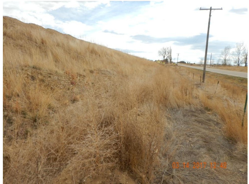
Photo 14. Photo taken from the northwest location, facing South. Vegetative growth makes it difficult to observe but a ditch and berm BMP has been installed around the perimeter of the location. Fill slope along the northwest corner does not appear to be stable. Appears portions have shifted and settled out over time. Additional stabilization may be required.
