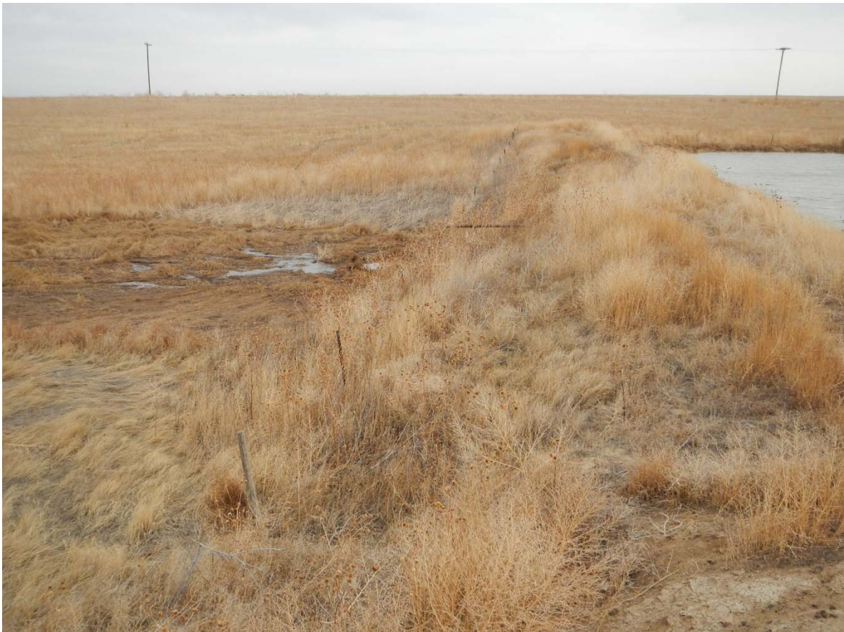
View east at surface discharge outfall.
