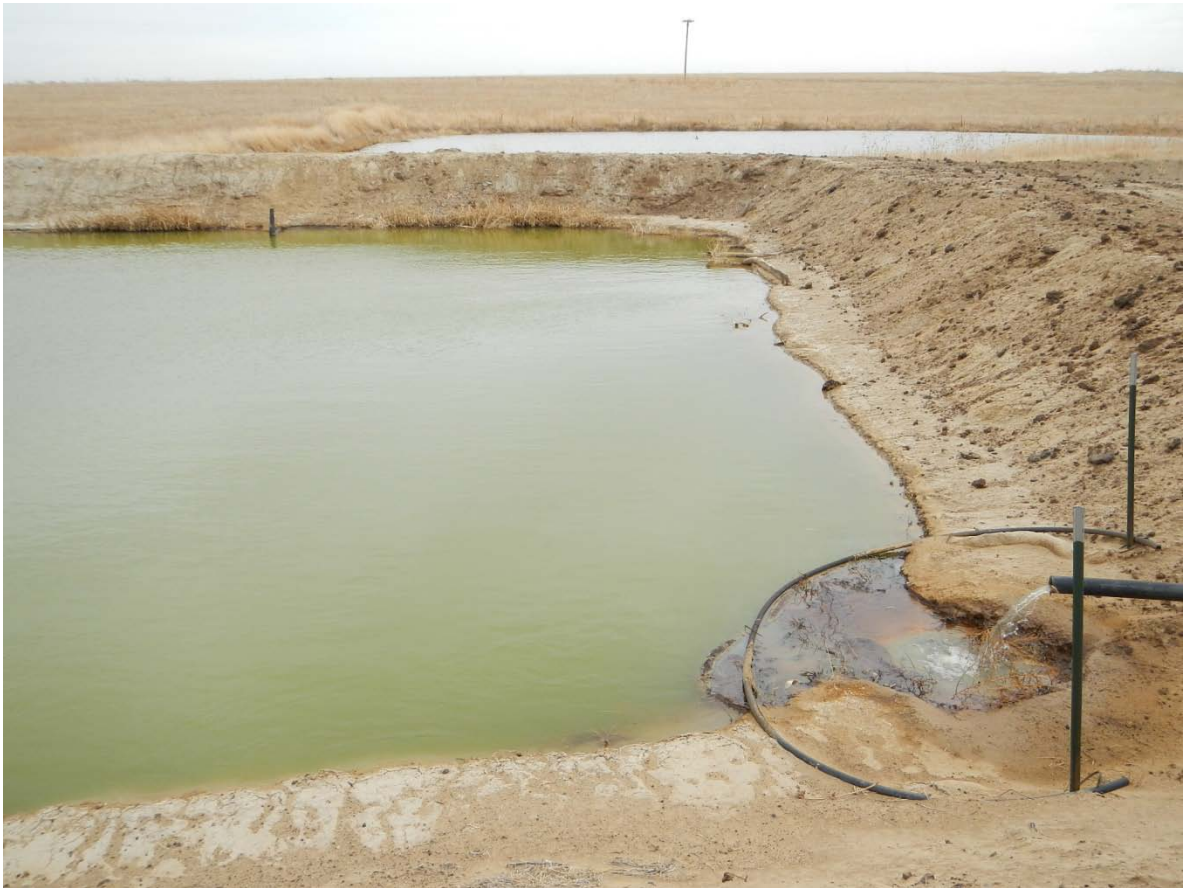
View east from produced water tank outfall (center pit).
