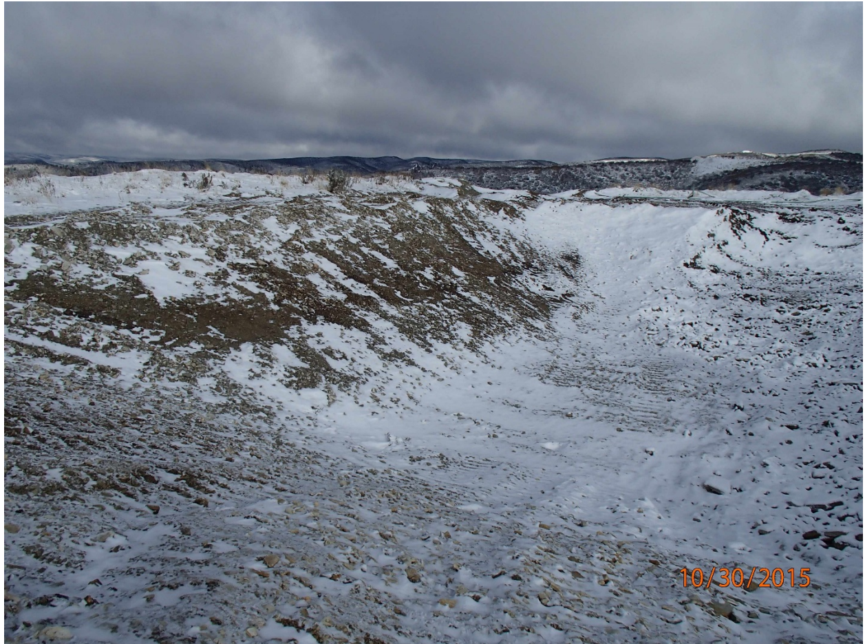
Subsoils post additional excavation on eastern side wall.
